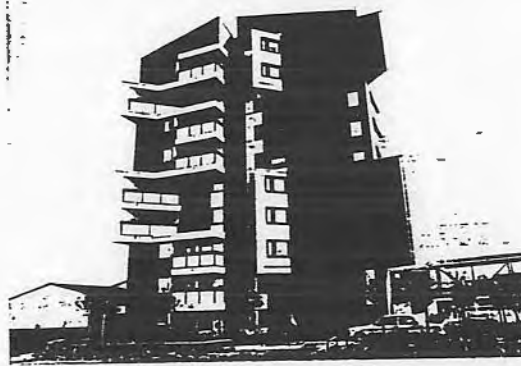
The north side of the 10-story apartment building. The bridge connects the "tower" to the low-rise apartments for the elderly
