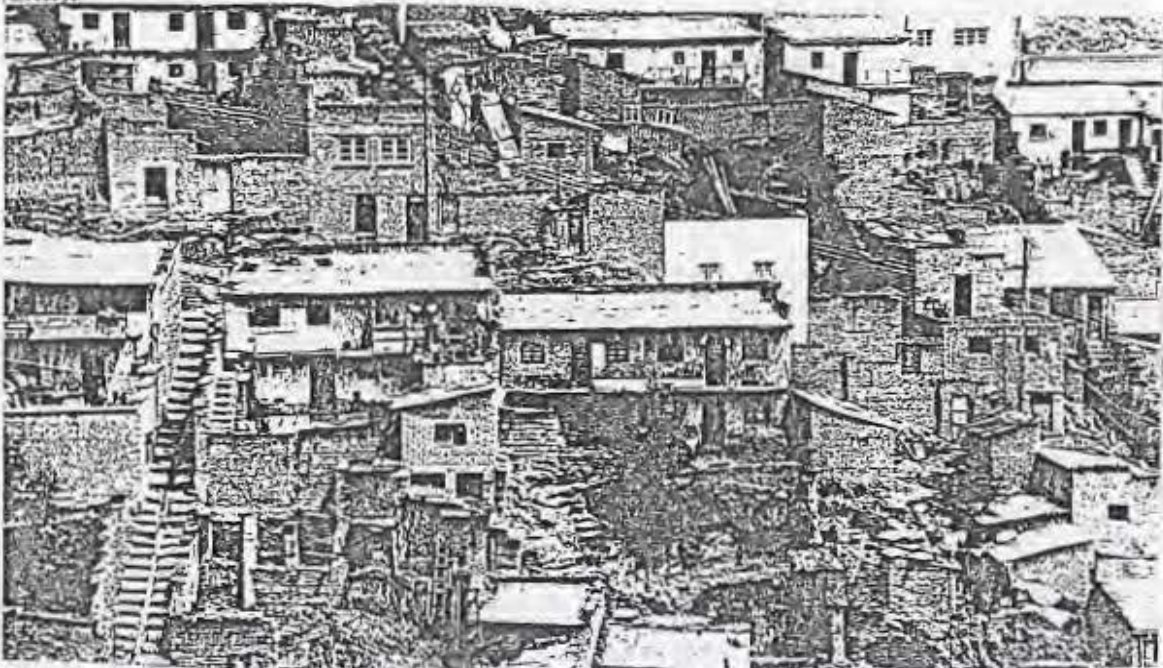
La Paz, Bolivia (1976). All these communities are firmly settled; the construction is of durable materials; many dwellings show an advanced state of completion. In La Paz, different stages of development can be seen; piles of bricks are everywhere, some dwellings have unplastered walls but in others walls are finished; steps are carved into the ground, but there is a stair in concrete, with a drainage channel in the center; poles and lamps for electricity and street lighting are already installed. Invariably, community improvements are the result of their own efforts. (Photos: B. Tokman, E. Popko, B. Kazimee, G. Gattoni.)
