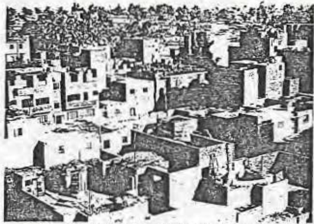
Fig. 14: Aimas and high density housing in the south of El Heker legalized housing.
