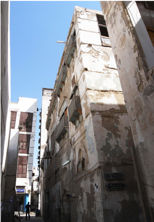
Fig. 1 Al-Nawar house in Old Jeddah, North facade, street view.
