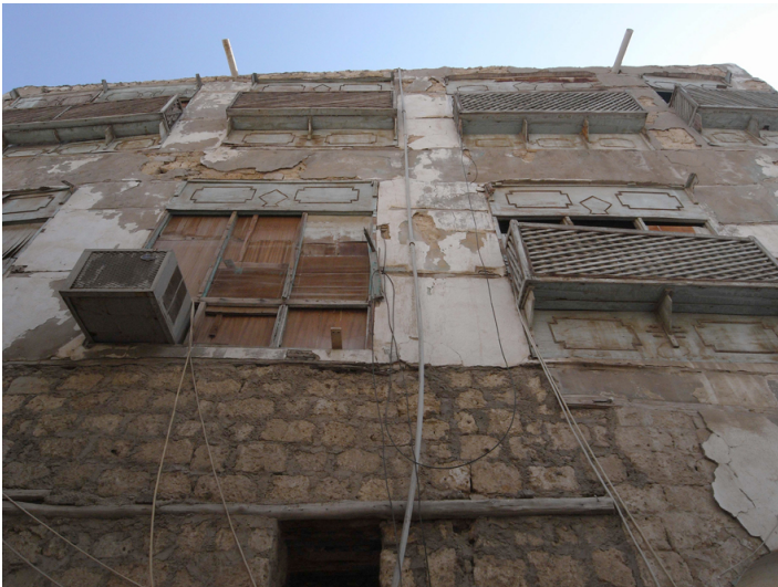
left: Fig. 19 North facade of the building, with characteristic wooden layers and large openings. A part of the wall is a recent reconstruction. Air-conditioning, water and electricity supply is added from outside. right: Fig. 20 Pilaster in the Northwest of the South part, leaning into the courtyard.
