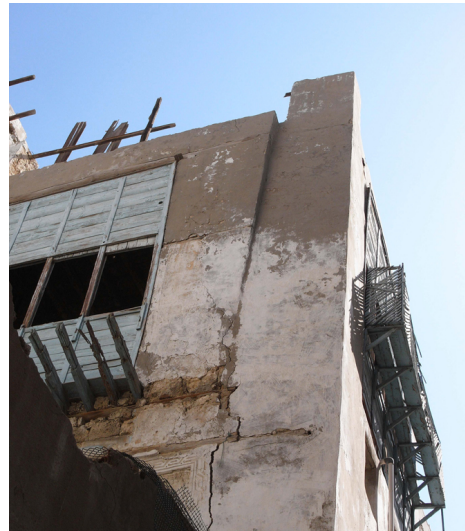
left: Fig. 19 North facade of the building, with characteristic wooden layers and large openings. A part of the wall is a recent reconstruction. Air-conditioning, water and electricity supply is added from outside. right: Fig. 20 Pilaster in the Northwest of the South part, leaning into the courtyard.
