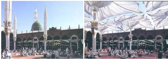
Figure 8: The courtyard of the Noble Prophet Mosque covered with sunshades during the daytime and could be folded in the night.
