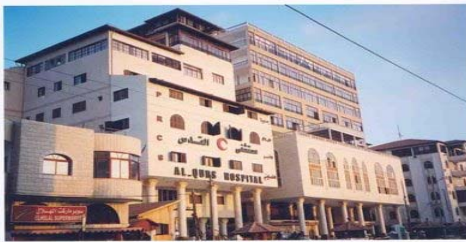
Figure (9) Alquds Hospital
