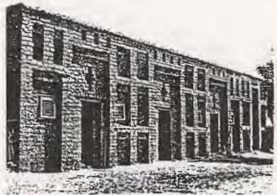
Fig. 18a Protruding and Recessing bricks are designed in Attractive motifs to give as much shades as possible in the Mali House Architecture.
