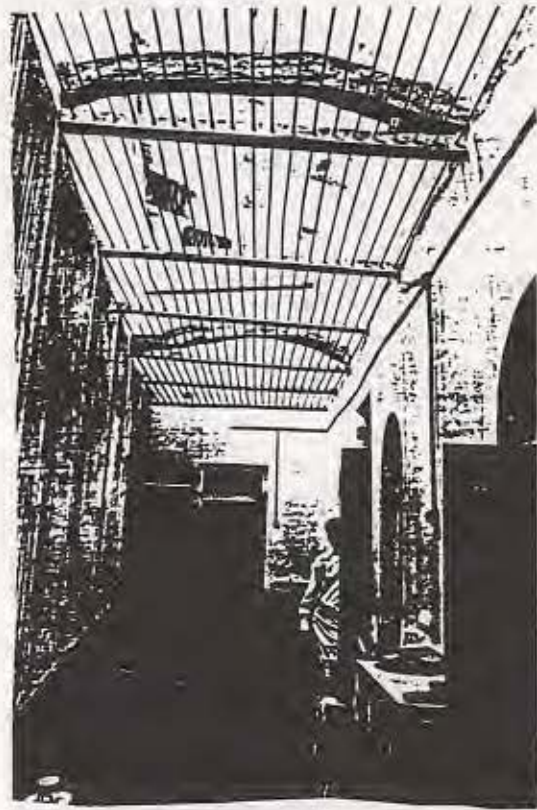
Fig. 14 Long narrow rooms in the EW Axis, all wind catchers have a metal grate to prevent entry into the house.
