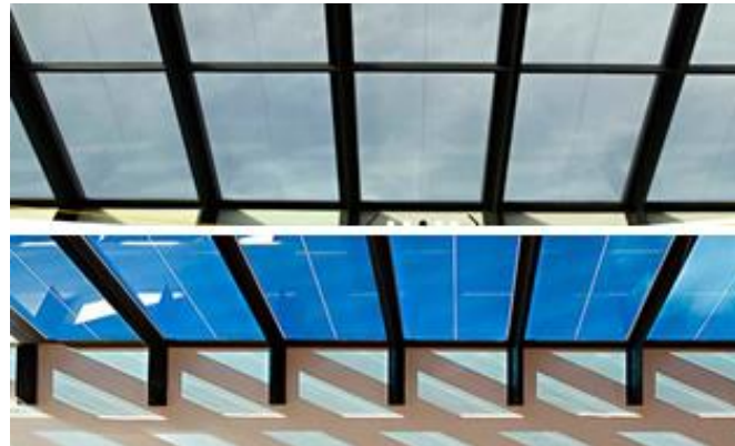
Fig. 10. Skylights ceiling from electro chromic glass, which is smart, dynamic, electronically tint able, control the level of daylight, and heat gain, as well as it reduces energy consumption (Sage glass, 2019)
