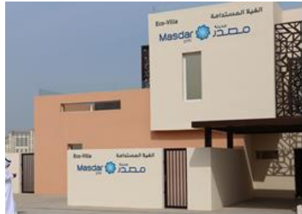
Fig. 15. Eco-villa model in Masdar city which consumes 100% Renewable Energy, and less than one quarter energy than the traditional villa (Masdar city, 2019)
