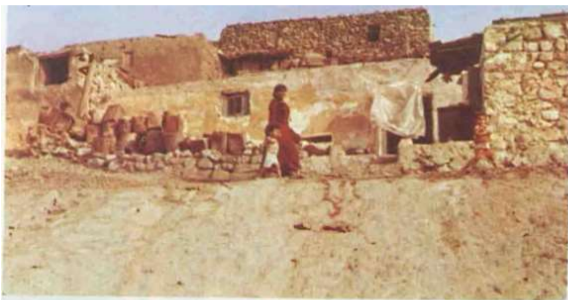
The rural character of life and building modes could be clearly recognized in areas of informal housing. This shows that most of the occupants have originally migrated from the country-side to the city.
