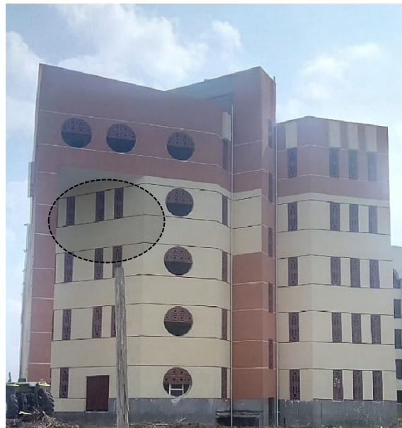
Fig. 8 a multi-story building with lattice windows-Tanta university, Egypt
