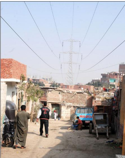
Fig(9): High voltage cables penetrating a village in Geiza, Egypt -www.masress.com
