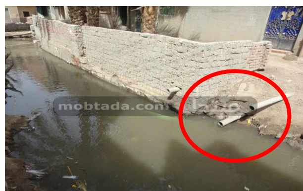
Fig.3 Household outlets discharging raw-wastewater into waterbody in Tersa, AlFaium.
