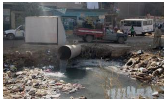
Fig.5 Left: Effect of wastewater discharging on total dissolved solids of groundwater in Egypt (1994 -2012) – Right: Wastewater treatment municipal plant in Mehallet Hassan, Gharbeya, discharging poor treated wastewater into open drain. Source: Easa & Abou-Rayyan, 2012.
