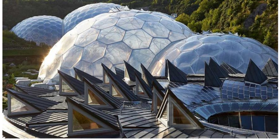
Figure 1 The Eden project at Cornwall-Uk source edenproject.com
