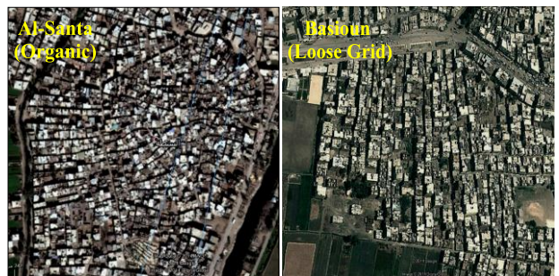
Fig(7): Two main street patterns in rural Egypt: Organic in Al-Santa and Loose grid in Basioun
