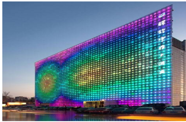
Picture (5): The elevation of the glasses curtain wall that is developed by adding photocells to glass sheets near Beijing Olympics – China 2008.
