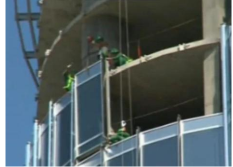
Picture (6): Closer picture for fixing and installing one unit of the glassed curtain wall used in the Skyscraper “Khalifa Tower” Dubai-UAE 2010.
