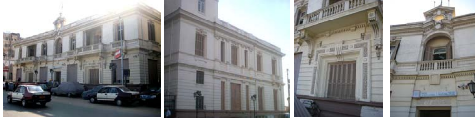
Fig.12. Façades and details of "Bank of Alexandria" after restoration.
