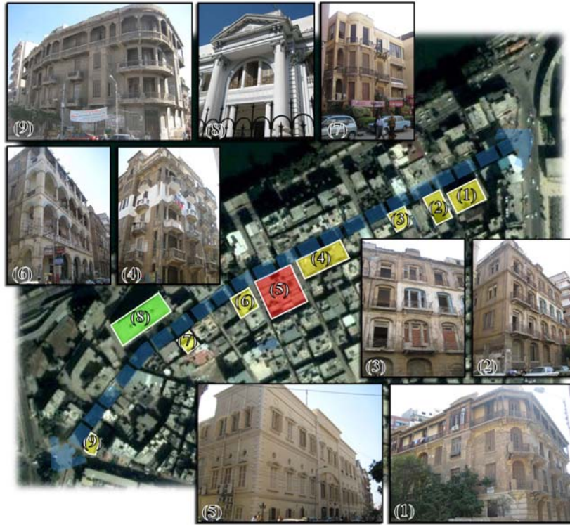
Fig.15. Fareda Hassan St. the buildings (1),(2),(3),(4),(6),(7),(9) are private residential, (5).Mansoura Court previously “Mohamed Ali Palace” , (8). Mansoura secondary school for girls.
