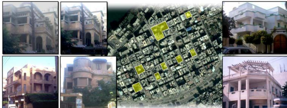
Fig.18. Torel Neighborhood. Some remaining villas.
