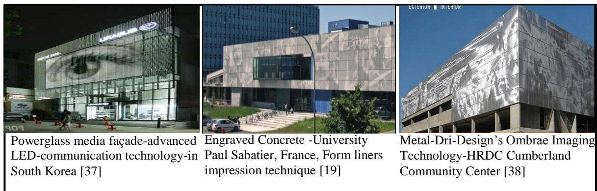
Fig.10. Diversity of technologies and building materials for the perception of facades with 3D images. The perception of drawings is varied according to the illumination, shades and building vision angle, Source: [19], [37] & [38]
