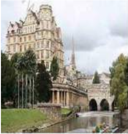
Pultiney Bridge River
