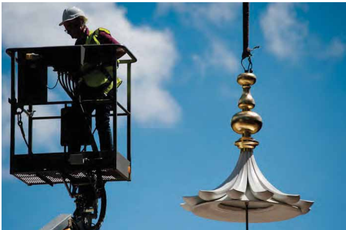
Fig. 207 - New dome finial being placed
