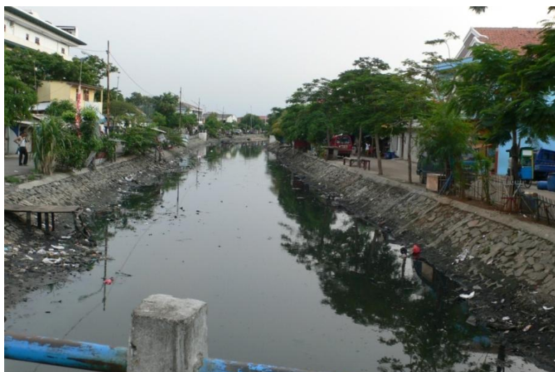
a: low-lying places to serve as water retention areas Source: Taken by the researcher in Jakarta, Indonesia, 2013 Figure 3-1: Selected examples for global adaptation measures
