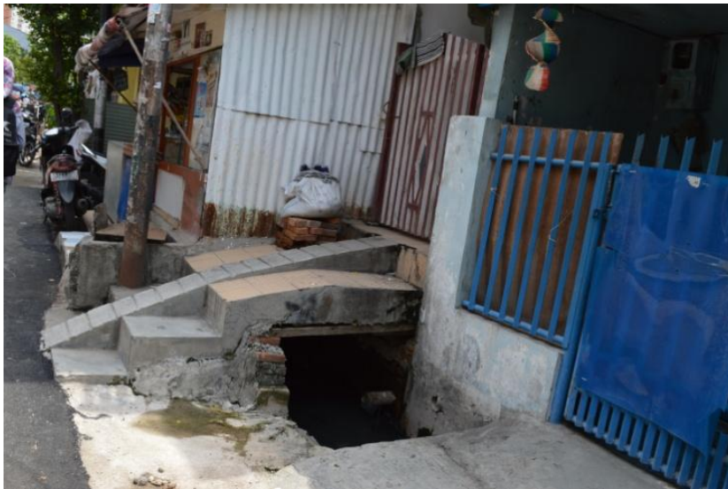
d: Rain drainage system combined with elevated house Source: Taken by the researcher in Jakarta, Indonesia, 2013
