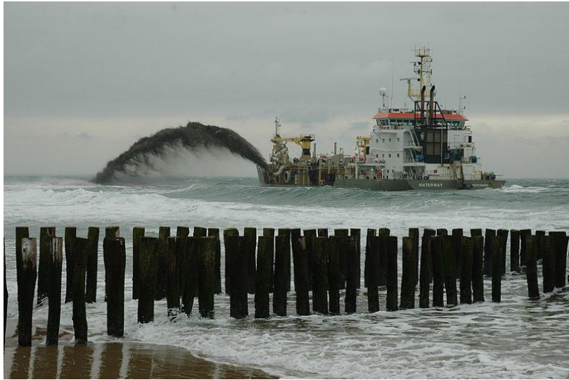
b: Dune reinforcement on the Dutch coast
