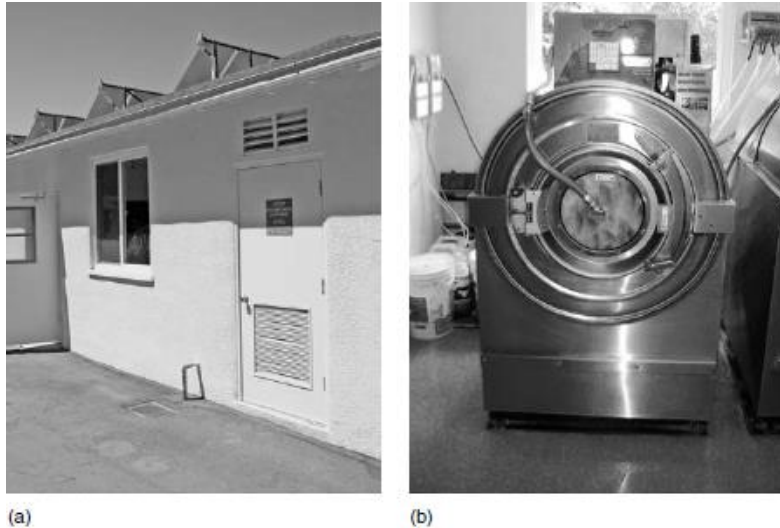
Figure 68 A laundry facility utilizing treated water with commercial size washing machines: (a) facility building with a notice of treated water use on the door and (b) laundry machine (Asano, Burton, Leverenz, Tsuchihashi, & Tchobanoglous, 2007)
