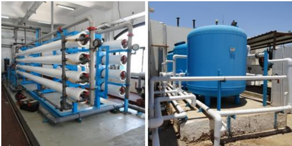
Figure 116 Left: Reverse Osmosis filtration tubes, Right: Sand filters (Photographed in Movenpick Naama Bay resort by the researcher)
