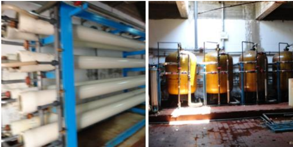
Figure 115 Left: Reverse Osmosis filtration tubes, Right: Sand filters (Photographed in Hilton Sharm Dreams resort by the researcher)
