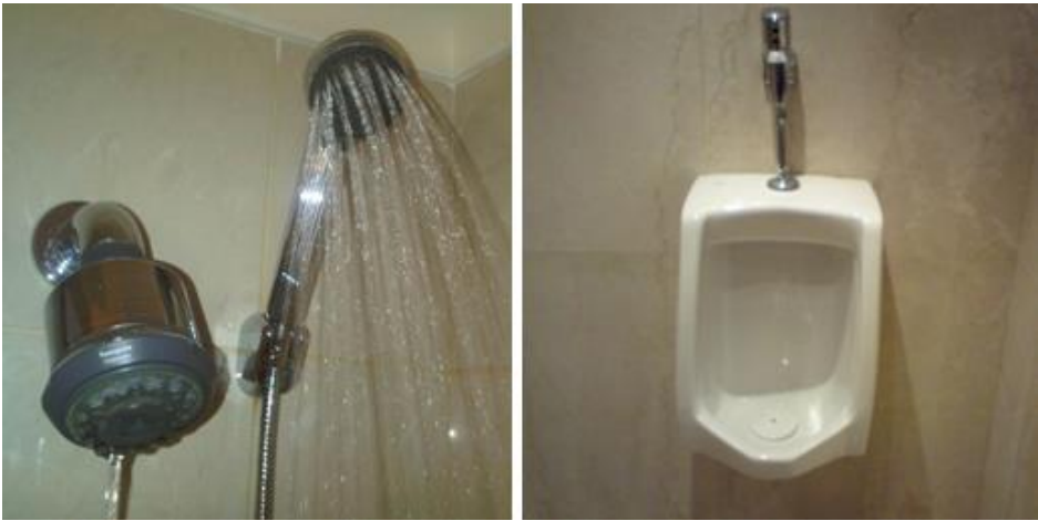
Figure 125 Left: Showerheads (water-rated), Right: Infra-red urinals (public bathrooms) (Photographed in Movenpick Taba resort by the researcher)
