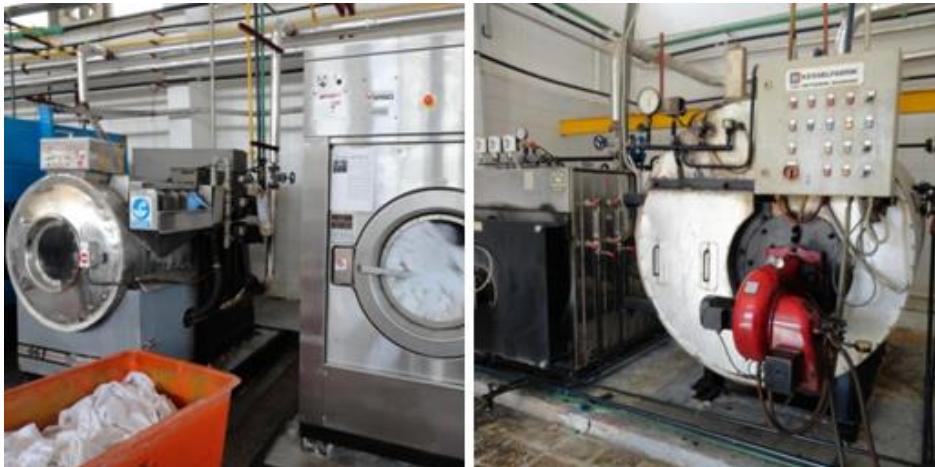
Figure 132 Left: Clothes washing machines, Right: Steam boiler for dryers (steam trap) (Photographed in central laundry service shared between Hilton Taba & Nelson Village resort and Movenpick Taba resort by the researcher)
