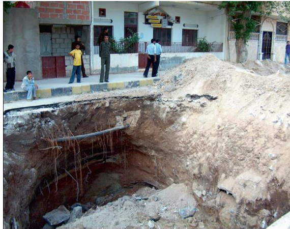
Figure 15 Sinkhole formed due to drawdown of the aquifer at Ras El-Ain, Syria (Pereira, Cordery, & Iacovides, 2009)
