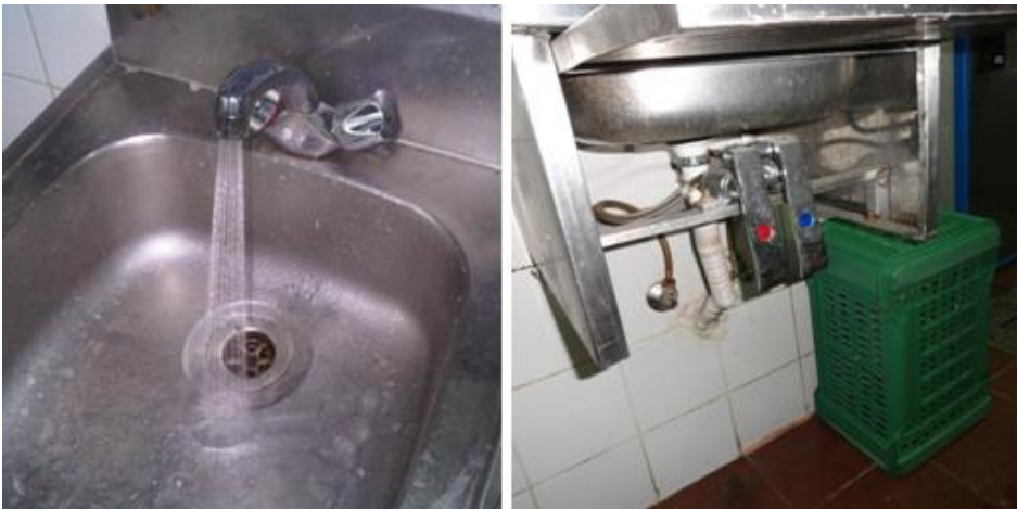
Figure 130 Left: Taps (flow restrictors used), Right: Pedal-operated taps (Photographed in Movenpick Taba resort by the researcher)
