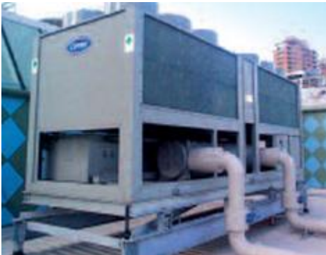
Figure 43 Left: Air-cooled chiller, Right: Schematic of ground source geothermal system (Corr, Adams, & Boynton, 2009)
