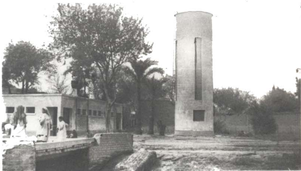
Water tower & washing places
