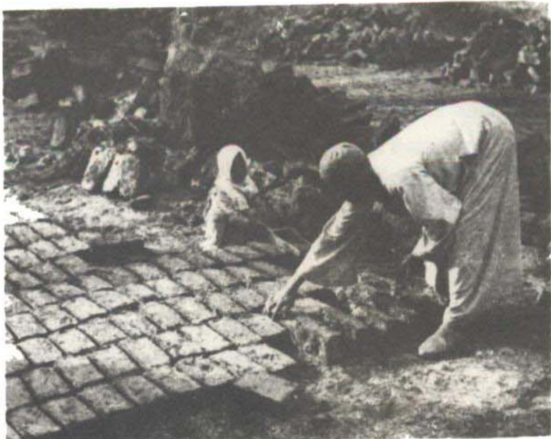
Drying out the mud bricks
