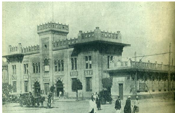
Figure 2-42: The original Pont Limun annex station.
