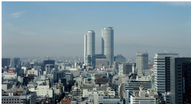
Figure 6-15: Nagoya Station, its towers seen from a far distance.
