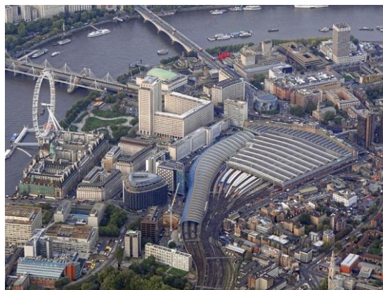
Figure 5-3: Bird-eye view of Waterloo Station, London.
