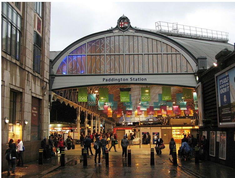
Figure 2-14: Paddington's current state of the façade.
