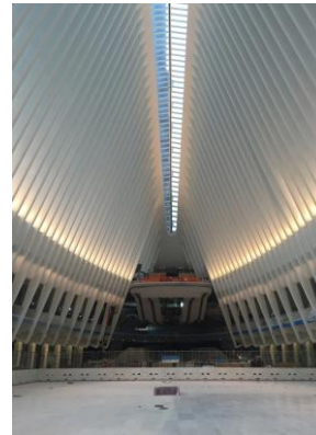
Figure 5-45: Interior of World Trade Centre Transportation Hub.
