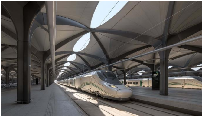
Figure 6-23: HSSR platforms covered by canopies.
