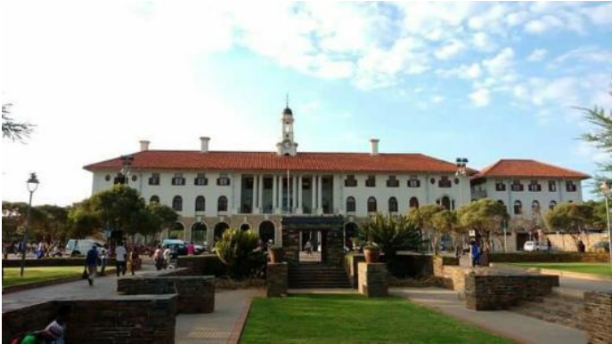
Figure 2-29: Pretoria Station, South Africa.
