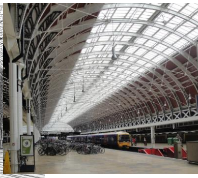
Figure 2-17: Paddington's train shed interior.
