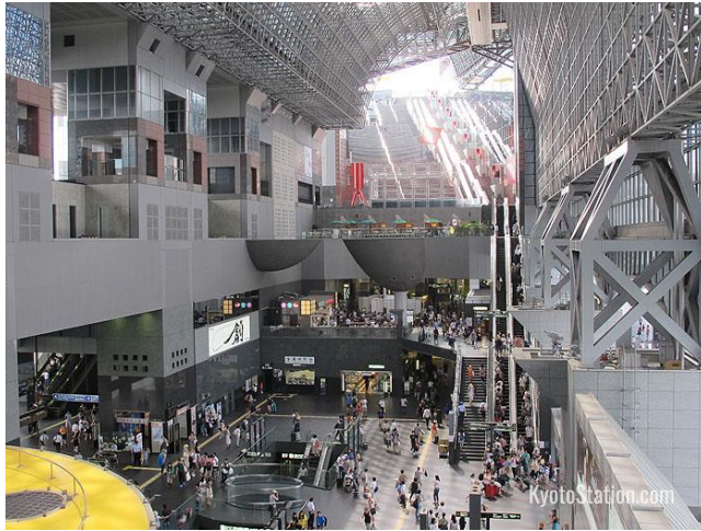
Figure 5-40: Central hall of Kyoto Station.
