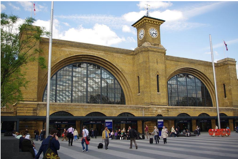
Figure 6-1: King's Cross station post-restoration.
