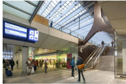
Figure 5-42: Roof glass plates vary light transmittance level by utilizing different solar cells patterns.
