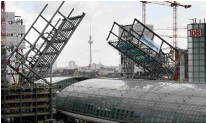
Figure 6-13: Lowering the constructed bridge above the main shed, Berlin Central Station.
