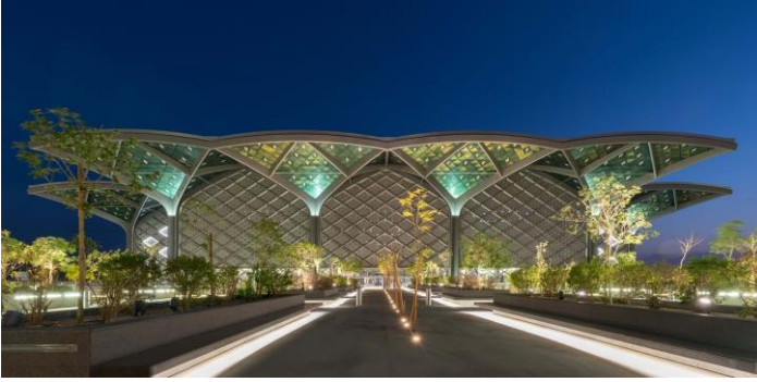
Figure 6-35: Exterior night shot of Madinah Station.
