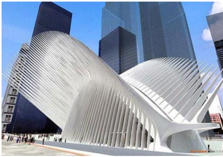
Figure 5-44: Exterior of World Trade Centre Transportation Hub.
