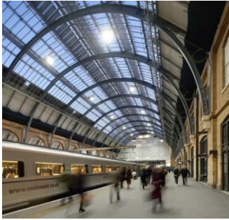
Figure 6-25: One of two steel & glass vaults over the platforms, Kings Cross.
