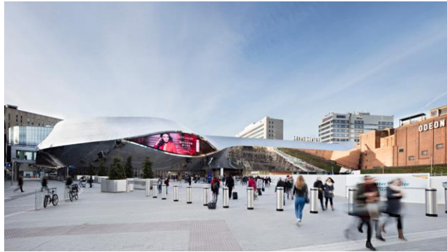
Figure 5-32: Birmingham New Street Station, UK.
