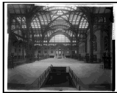
Figure 2-51: Penn Station's main concourse.
