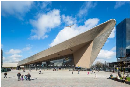
Figure 5-41: Grand entrance of Rotterdam Central Station.
