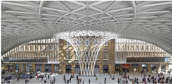
Figure 6-5: Radiating tree-form of west concourse, King's Cross.
