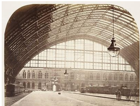
Figure 2-22: The south elevation before the completion of the Midland Grand Hotel, 1868.
