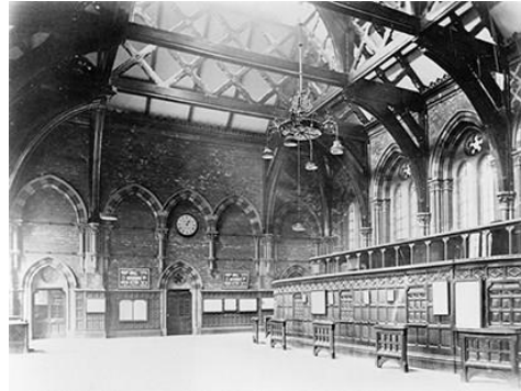
Figure 5-36: The St Pancras Station Booking Office in 1900, showing the original roof.
