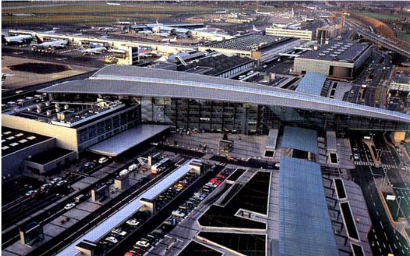
Figure 5-6: T3 and its station, Copenhagen Airport.
