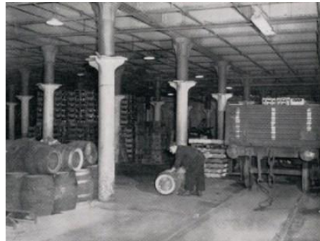
Figure 2-23: Hydraulic lift used for beer transport to the undercroft.
