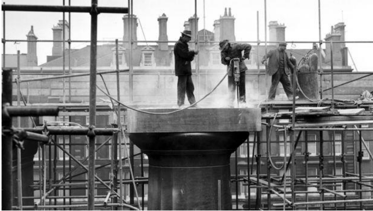
Figure 3-1: Euston Arch being dismantled, 1961.
