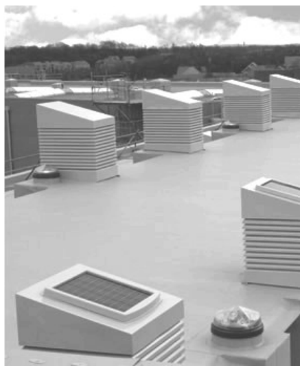
Figure 3- Wind catcher with polycrystalline solar panels for generating power, Hazeley School 24
