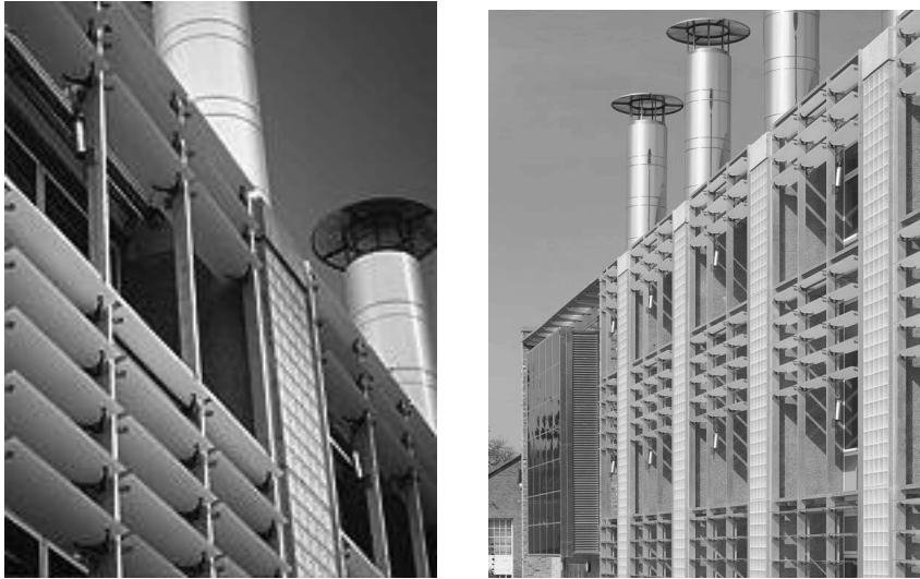
Figure 4- Applications for second glass louvers carrier system, BRE building, Garston 13
