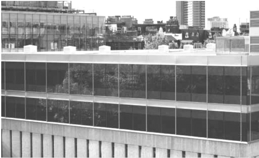
Figure 3- View of the Windcatchers from outside on the Imperial College library roof 34
