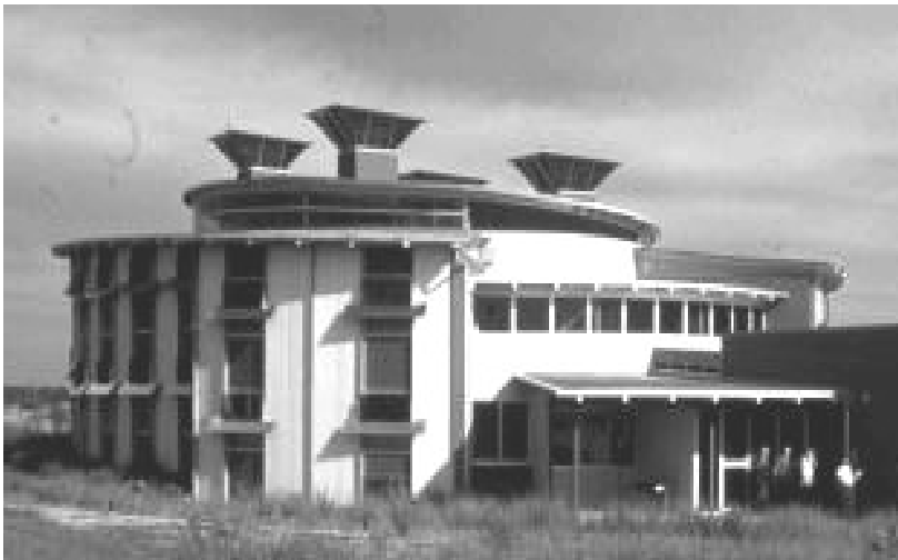
Figure 2- Passive Downdraught Evaporative Cooling, Dubbo Campus, Charles Sturt University 70
