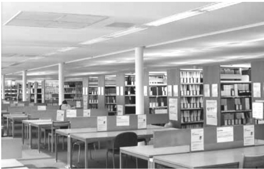
Figure 3- Interior view of the Windcatchers diffusers on the ceiling of the library 35
