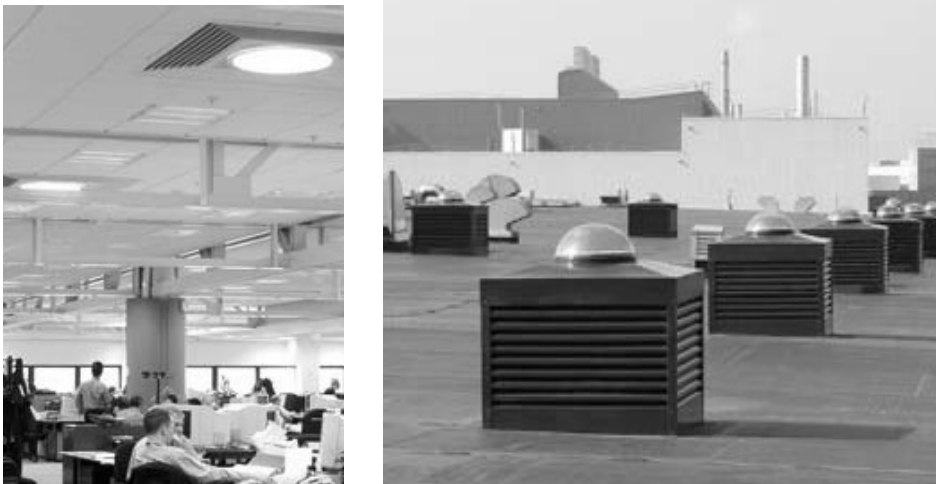
Figure 3- The solar-wind catcher system in BMW head offices 33
