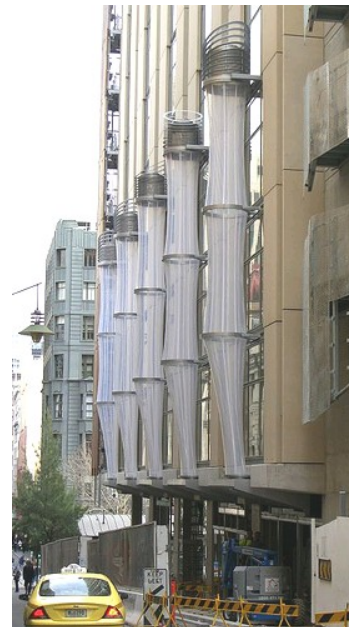
Figure 5- Chilled water runs through radiator coils to absorb heat gained from glass facade 14
