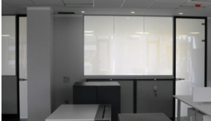
Figure 4- Application of switchable smart glass in corporate headquarters: when it is switched on (partial transmission for light) 69
