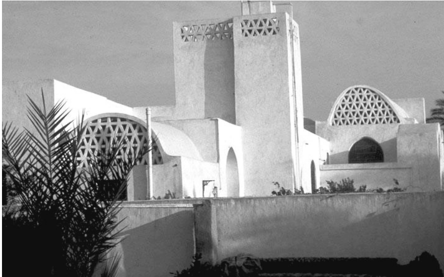
Figure 1-traditional sustainable architecture: Akil Sami House, Dahshur, Egypt 3 Example of Fathy's sustainable architecture: using local limestone and the courtyard with wooden pergola.
