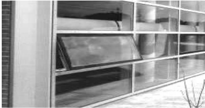
Figure 4- Movable aluminum mirrored louvers, Bruntland Center, Toftlund, Denmark 17
