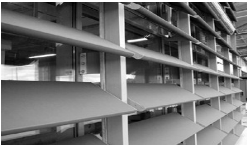
Figure 4- application on thermo hydraulic shading overhangs, the Johnston Press building in Sheffield, England 30
