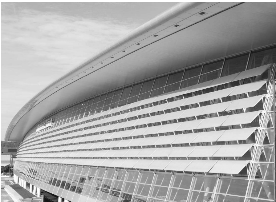
Figure 4- Automatically controlled metal louvers rotation with sun angels 0-90 degree 21
