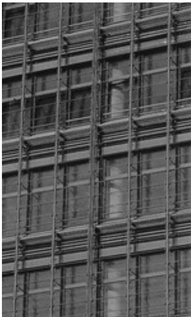
Figure 3- Wind driven natural ventilation in double skin façade (debis Headquarter postdamer platz) 69
