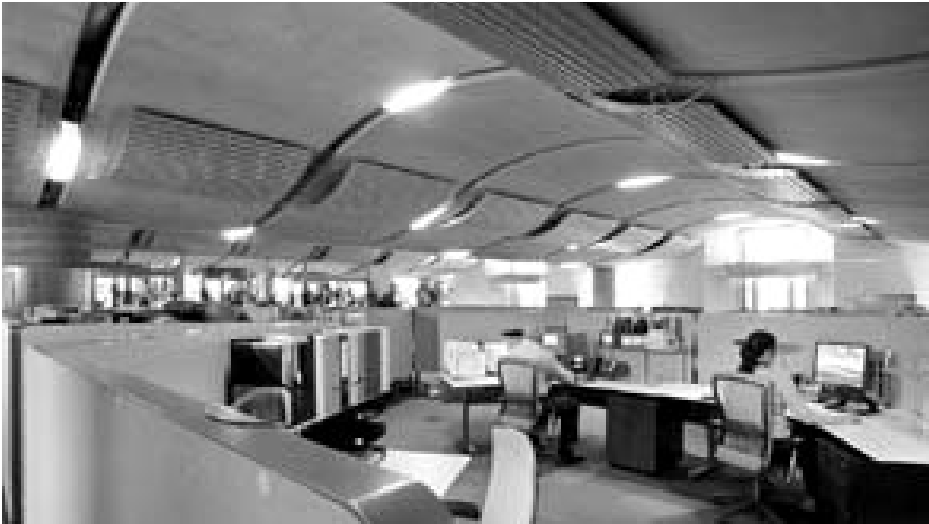
Figure 5- Interior view of vaulted concrete ceiling 9
