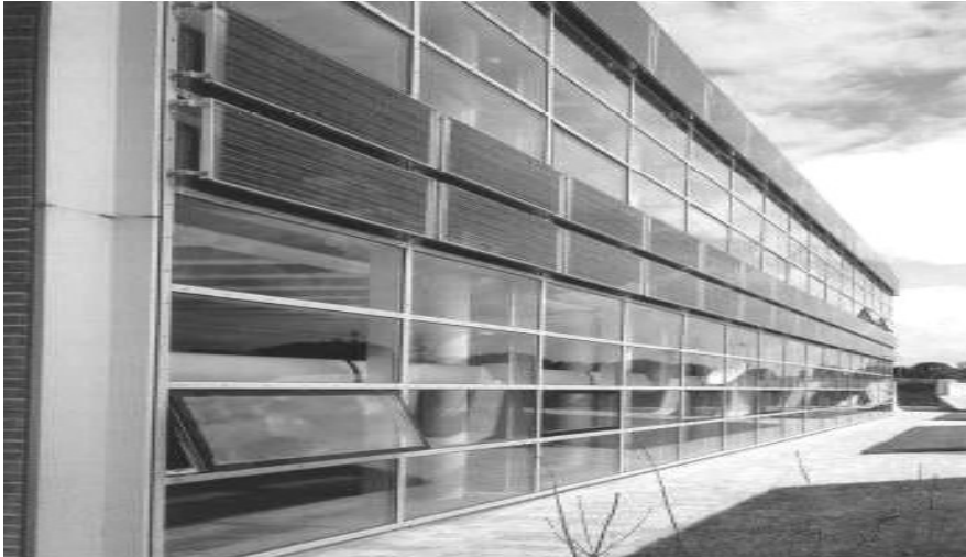
Figure 1- PV panels on Brundtland Centre facade, Tofitlund, Denmark, Krohn & Hartvig Rasmussen 19
