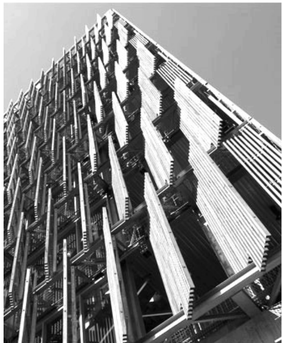
Figure 5- Exterior view, movable shading shutters on the western facade 25
