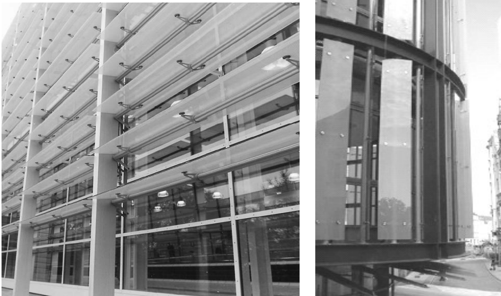
Figure 4- Applications for first glass louvers carrier system as horizontally or vertically, VW AutoCity, Germany
