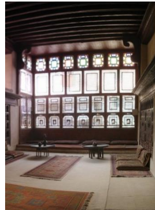
Figure 1.40 – Indoor space with full height façade of mashrabiya with two different patterns, for supplying and extracting air through same opening 2
