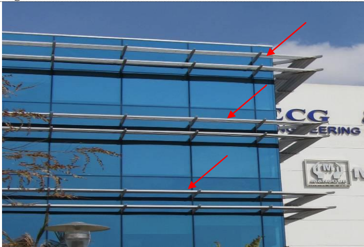
Figure 4.11: Louvers on South, East and West Elevations
