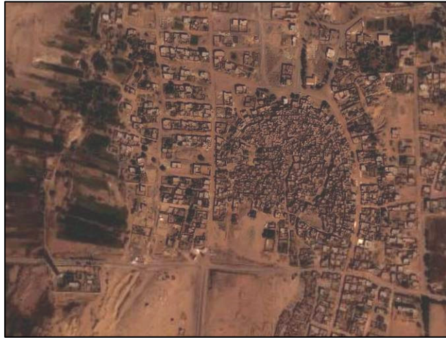
Fig.8-10: Vernacular village of Balat in Dakhla with a new extension
