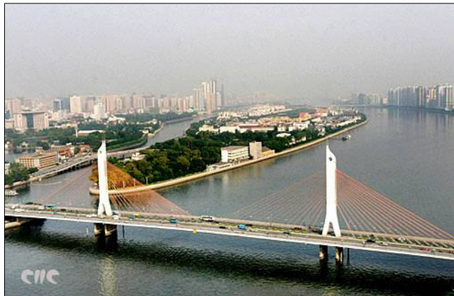
Fig: 3-22: The Haiyin Bridge linking Shenzhen and Hong Kong in the PRD
