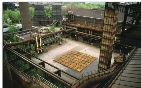
Fig. 3-14: Piazza-Metallica at Duisburg – Nord: Redeveloping Spaces in Emscher Park Source: www.upenn.edu/gazette/ , August 2007.
