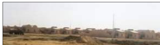
Fig.6-31: The demo project in the form of a planned settlement still deserted despite its completion.
