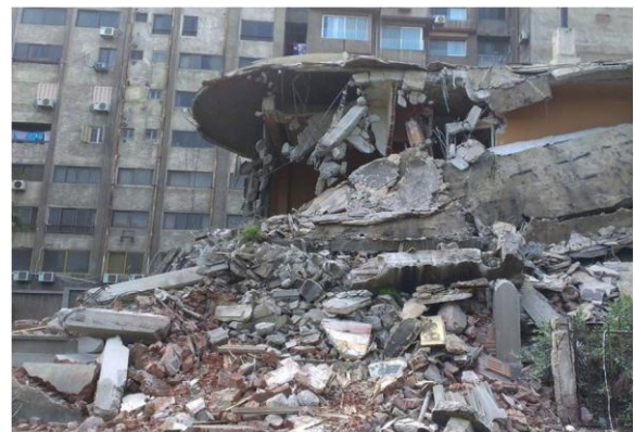
Figure 4-6: Villa "Aghion" after demolishing [75].
