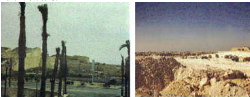
Fig 5.15 Shows works of stone along the coastal road in the north west coast
