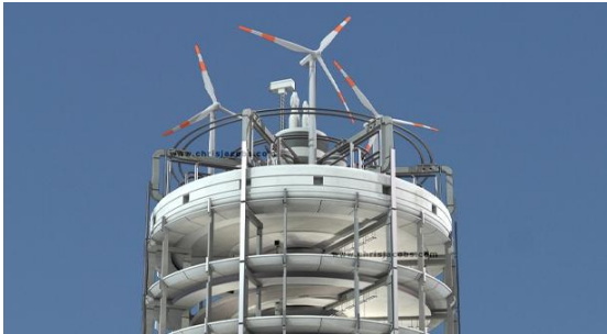
Fig.12 Horizontal axes machine located on a building
