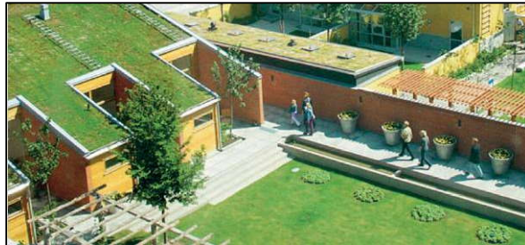
Figure (5-11) Roof gardens in Malmö
