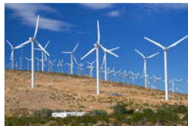
Figure (3-5) wind farm
