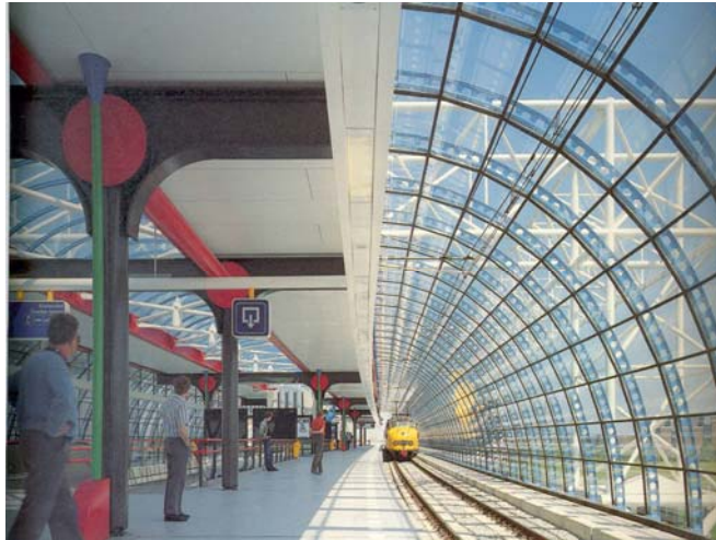
Fig (2.22) Platform shelter at Sloterdijk Station Amsterdam. [5]
