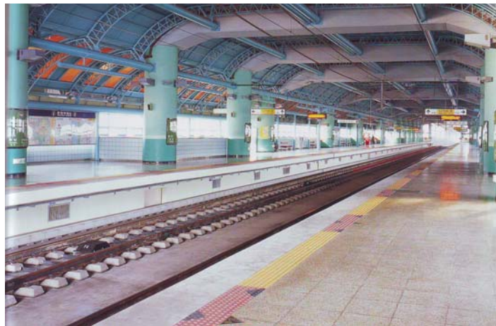
Fig (2.11) Identifying the edge of platforms with changes in texture and pattern is an important safety factor, Gyeongbokgung Station.[10]
