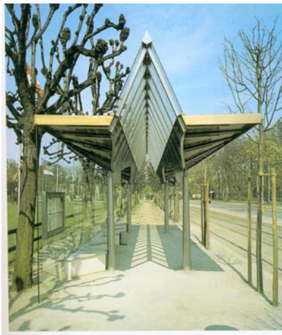
Fig (2.20) Street car station in Hannover, for the roof the architect used iroko wood in the interior, and copper plate on the exterior. The pillars are stainless steel and the bench is cement, with seats made of Corian acrylic resin. [3]
