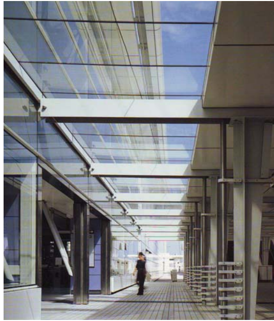
Fig (2.32) Skylight entrance to station concourse, Tung Chung Station, Lantau, Hong Kong. [8]
