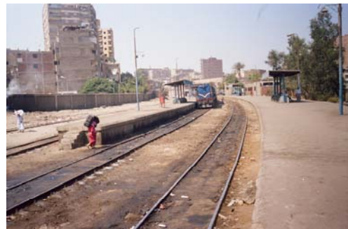
Fig (2.22) View of ENR station platforms and tracks
