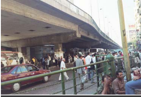
Fig (4.6) Congestion problem under 6 th of October expressway ramp
