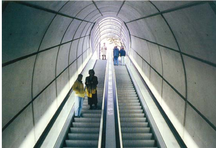
Fig (2.36) Queensland Rail's Roma Street Station, Brisbane, Queensland, Australia, Pedestrian entrance to subway
