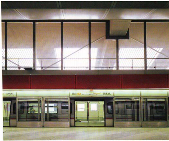
Fig (2.17) Platform screens reduce heat losses and provide safety for passengers.[8]
