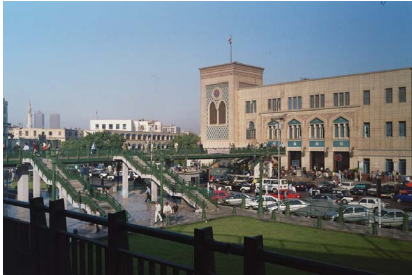
Fig (4.9) Ramses ENR station main entrance
