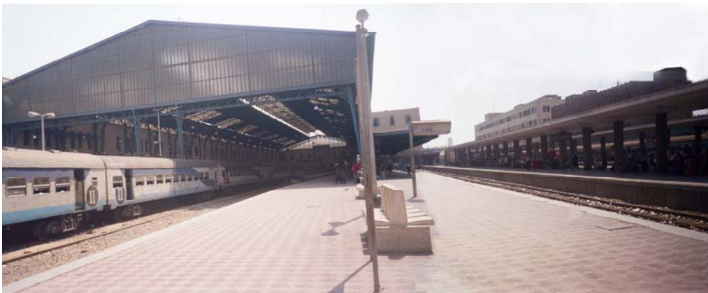
Fig (4.13) Rameses ENR station platforms and platform shelters
