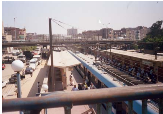
Fig (2.24) Metro Line 1 Station
