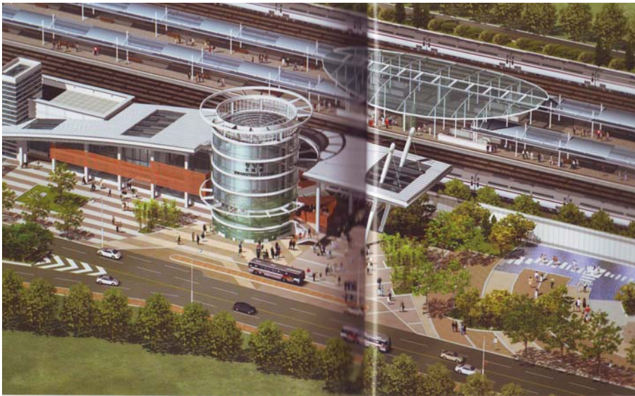
Fig (2.41) The use of light coloured materials for paving and planting shade trees reduce heat island effect as well as providing pleasant environments for users. Gwangyang Station.[10]
