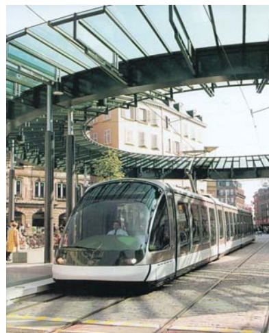
Fig (2.21) The circular glass shelter at the focus of place de l'homme de Fer at Strasbourg fort the streetcar which has become a viable ecological alternative to cars and busses. A central ring 35 metre in diameter was intended to give the plaza a pedestrian scale. [3]
