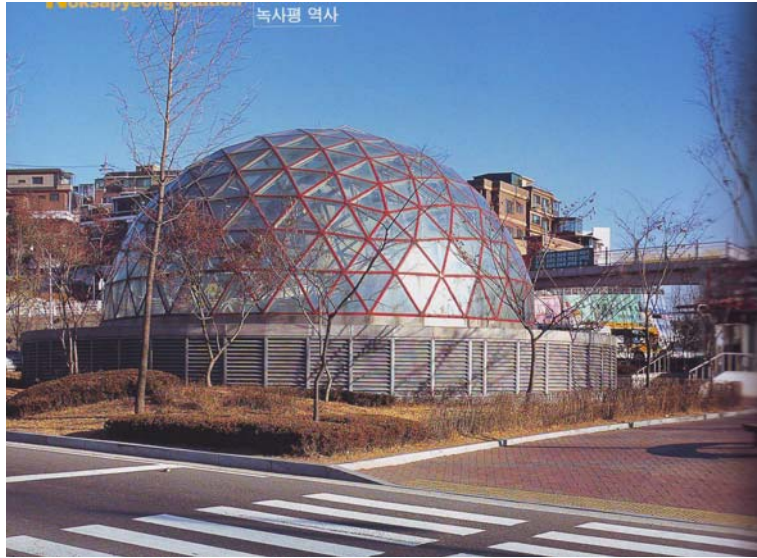
Fig (2.24) Dome exterior at Noksapyeong Station. [10]
