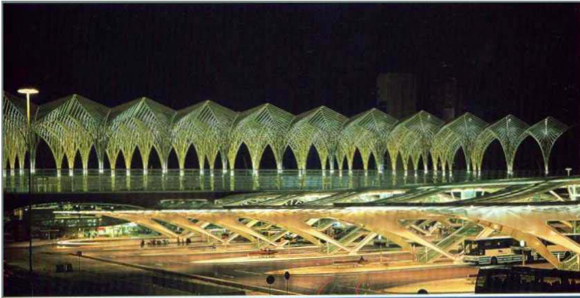
Fig (3.16) Overall view of Oriente Station with bus stations in foreground
