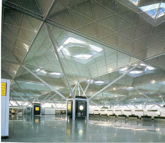
Fig (2.30) At Stansted, airport, the roof is a network of six by six metre steel tubes which inscribe modules having a repeated pattern. At the centre of each rectangle of three by three modules, is a tree of pillars, each bifurcating into four tubes and forming the node of a network. [3]
