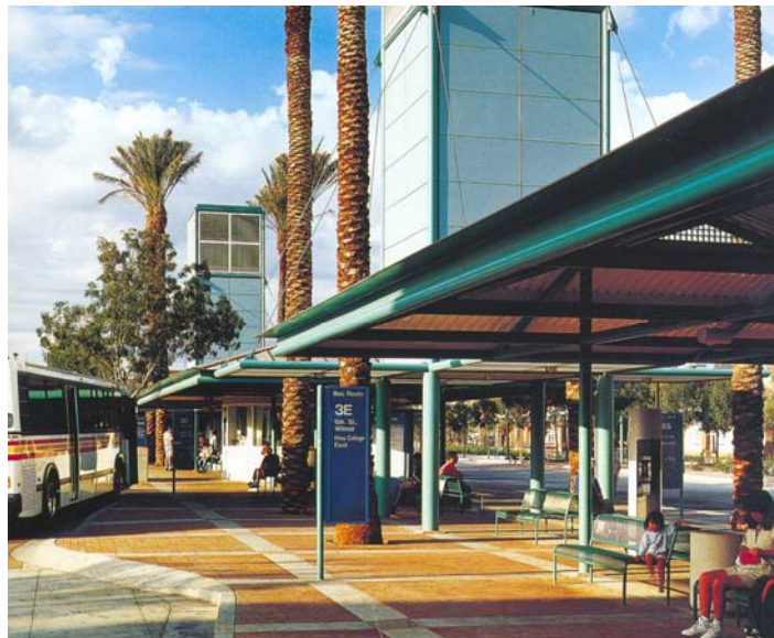
Fig (2.9) Shade canopy and neckdown at Ronstadt Transit Centre, Tucson, Arizona, USA, [18]
