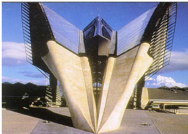
Fig (3.35) The building takes on the appearance of a bird, although a bird with a lighter, more ethereal appearance. The concrete roof over the platform area, almost at ground level. The steel roof traverses almost perpendicularly overhead. [3]
