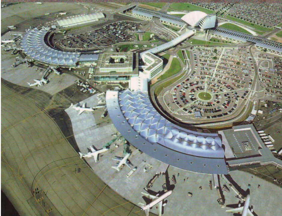
Fig (3.30) Lyon St Exupery TGV Station and airport terminal, aerial view.[1]
