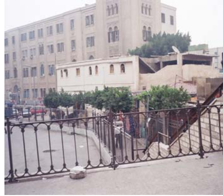
Fig (5.5) The buildings proposed to be demolished at the west of the ENR station
