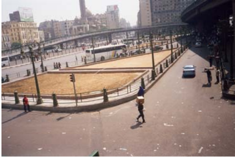
Fig (4.4) Slip road between Ramses street and access ramp to 6 th of October expressway and vacant area of the removed statue
