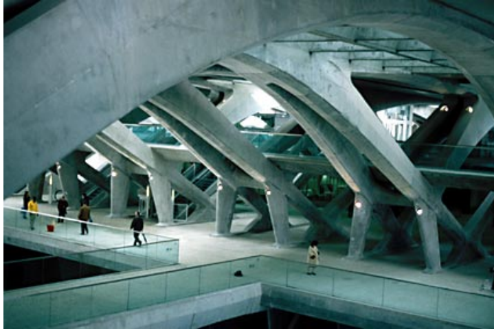
Fig (3.17) pedestrian walkways and the glazed canopies that are positioned as ribs, parapets are made of glass. [30]
