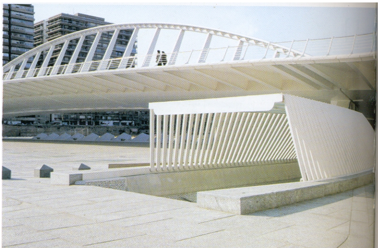
Fig (2.33) Treatment of the subway opening, Almeda bridge and subway station in Valencia. [8]
