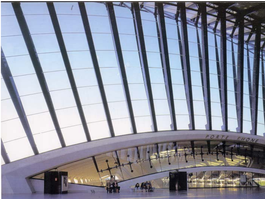
Fig (3.38) View of the access to the platforms from the lobby. Two roof components intersect over the hall .[3]
