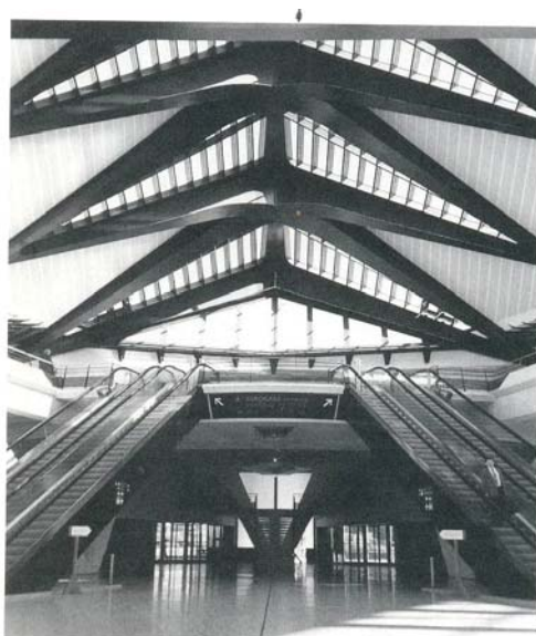
Fig (2.29) At Lyon St. Exupery Station, the escalators ascend towards the light from a large column free concourse. Space, light and expressive structure provide the means by which travelers are guided through the station. [5]
