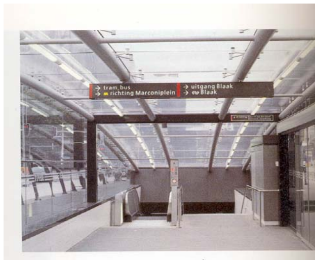
Fig (2.35) Roof canopy, Rotterdam Blaak Metro station, one of the functions of walls and roof canopies of underground stations is to pull light down into subterranean courses. Curved ceiling is particularly useful in this regard. [3]
