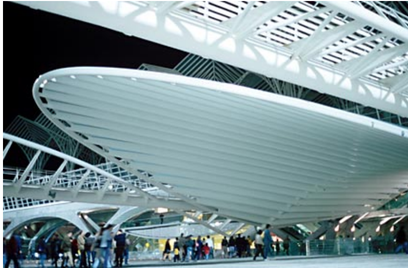
Fig (3.19) concourse area, Oriente Station [30]
