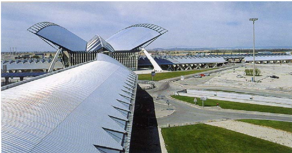
Fig (3.34) Lyon St. Exupery TGV Station, view of roof.[3]
