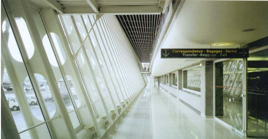
Fig (2.26) At Point a Pitre airport, Guadeloupe, the patterned metallic exterior facing covering windows of the large upper-level halls acts to filter and reflect sunlight, creating ever changing shadows on the floor throughout the day.[3]
