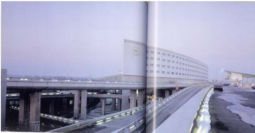
Fig (3.46) The hotel has been built along the axis of growth of the airport. [3]
