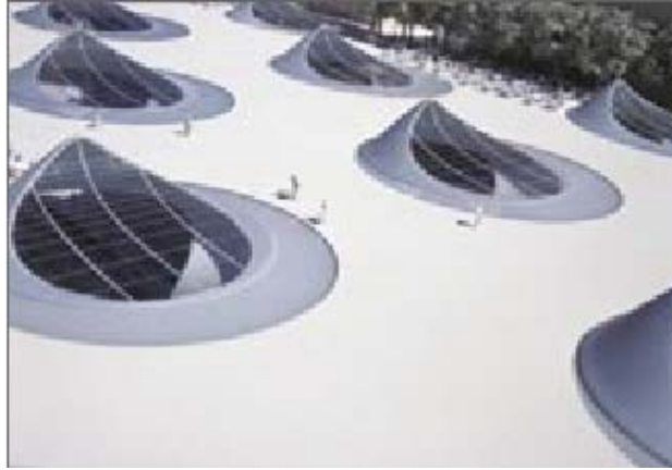
Fig (3.15) The surface-penetrating 'lighteyes' are the key characteristics of the design of the load bearing structure. [34]
