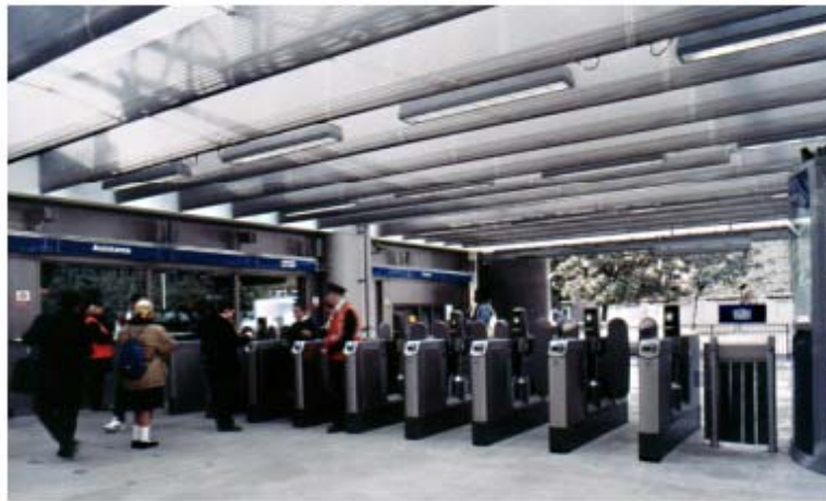
Fig (2.23) Ticket hall gate line at Bermondsey Station, exploiting natural light to create a clear special experience and a legible route between platforms and main station entrance (the station is covered by a translucent roof which allows sunrays to reach the rail platforms beneath). [12].
