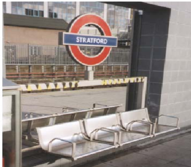
Fig (2.44) At Stratford Station, elaborate finishes with fire hazard potential are avoided and durable uncoated constructional materials like concrete, glass and stainless steel are very simple and should feel as right in 50 years as it is now[12]
