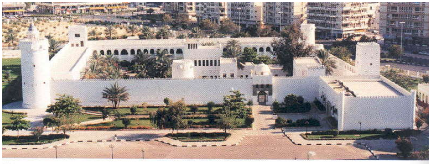
Figure 2a: Square enclosure with two diagonally placed towers ( Qasr Al-Husn in Abu Dhabi).
