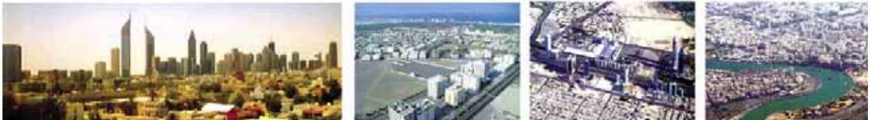
General views show the new urban development of Dubai city
