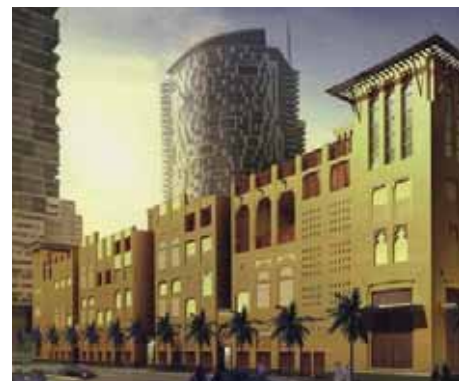
Fig. (6.22) Expression of regional architecture are shaping some emerging development in Abu Dhabi-UAE.
