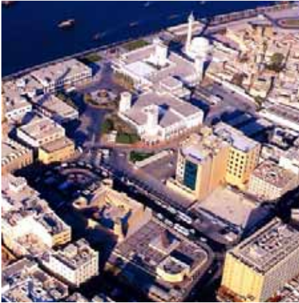
Fig. (6.27) The Al Feheidi Fort Dubai (built in 1799 and restored in 1994) is an good example of careful restoration, but isolated from its surroundings.
