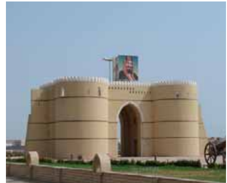
Fig. (6.35) Jeddah, the reconstruction of old city gate is a typical monumental work to enrich the city skyline and providing it with a historical dimension.
