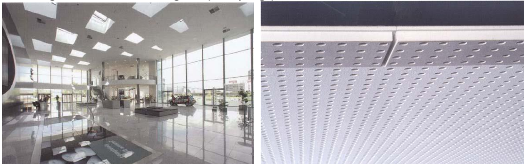
Figure 3.47 The European headquarters of Hyundai Motor Europe in Offenbach, Germany, is lined with air-purifying plasterboard panels.
