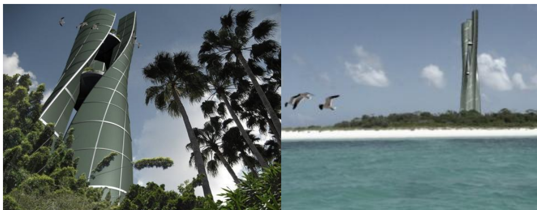
Figure 4.19 NVS tower, external view.
