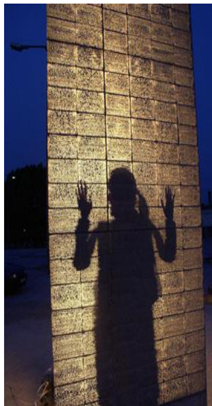
Figure 3.31 Transparent concrete Europe Gate, Komárom, Hungary.
