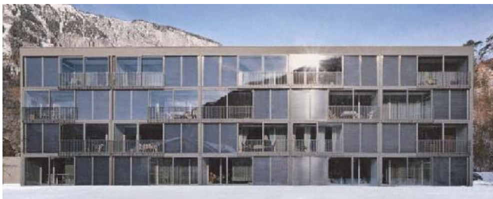
Figure 3.36 The south-facing glazing of a residential building, Swiss Alps.
