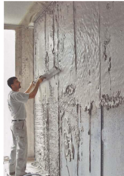
Figure 3.46 PCM plaster applied on Interior walls provides thermal insulation.
