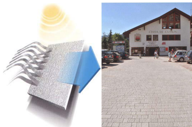
Figure 3.48 Concrete paving panels with photo catalytic air purifying properties used as a design element in a car park. Source; Sylvia Leydecker, 2008
