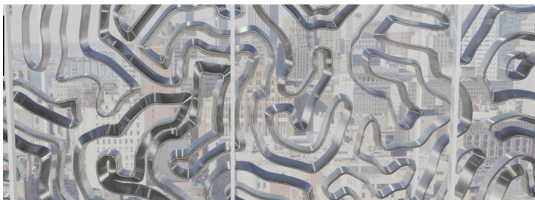
Figure 3.79 Homeostatic façade from inside.
