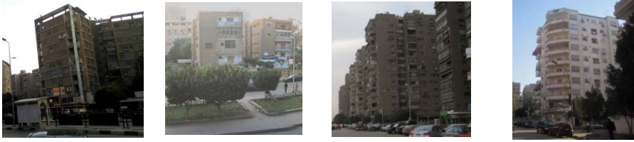
Figure 3-110 Building types in the International Garden area i
