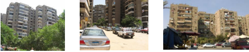
Figure 3-33 Building types in Al Tawfik area i
