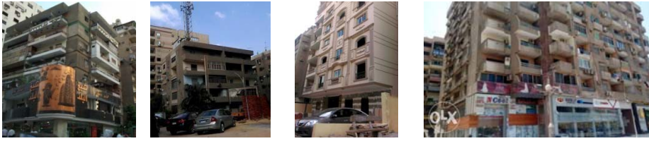
Figure 3-5 Building types in First Area i
