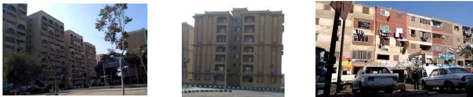
Figure 3-106 Housing levels in the 10 th Neighborhood area iv
