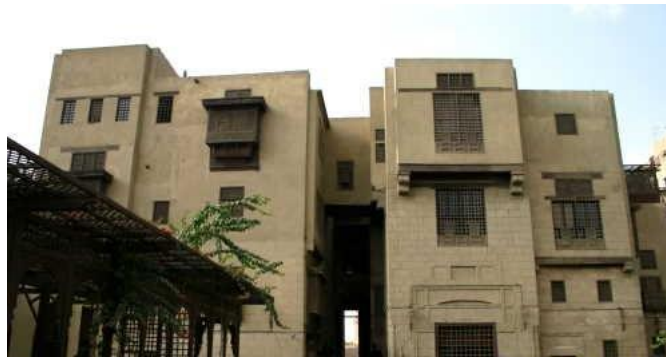
Figure 14: Bayt al- Kritilya shows the architectural characteristics of Islamic houses; the height of which is 2-3 floors, the solid facades and the woody windows with the work of the 'Mashrabya' [33]
