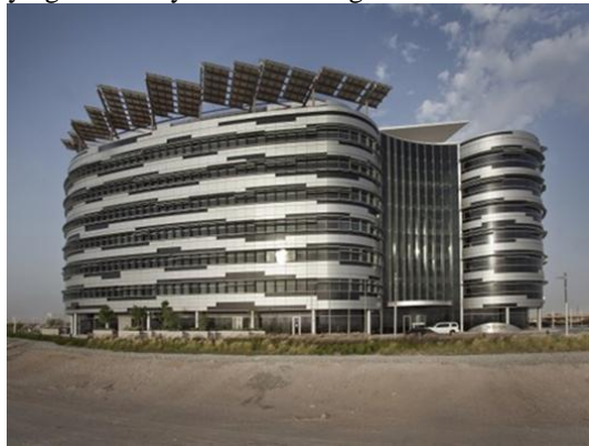
Fig (2): PV System on the Rooftop of Headquarters Building for the International Renewable Energy Agency (IRENA), Abu Dhabi, UAE, [7].
