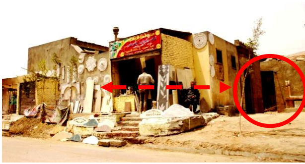
Fig.(45) Shows a small informal workshop for decorative plastering and gypsum forms standing right next to a graveyard that is exposed and located directly on the main road (Nasr st.)
