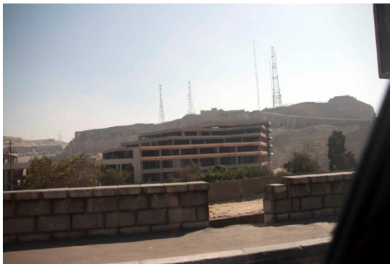
Left : Fig. (72) Major Project , that belongs to the late business man Mohammed Nosseir, stands on the other side of the Citadel had been stopped by HOUH. It shows how the NOUH is empowered by law to stop any activities that harm the historic urban areas. This is a clear example of how different governmental authorities act against each other. This project must have had an official permit from the governorate of Cairo before it was built. Photo taken by researcher
