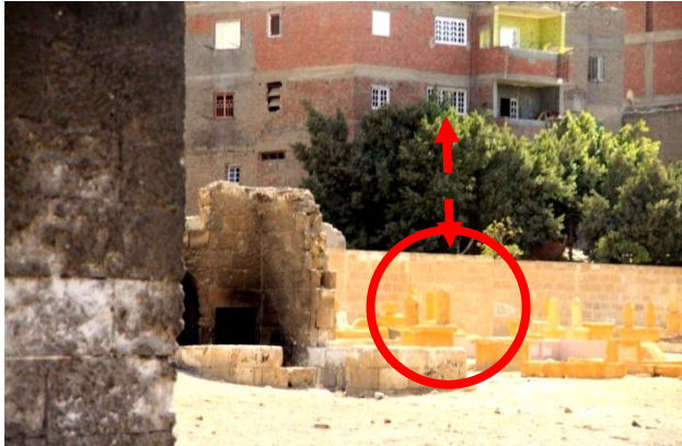
Fig. (47) Is a photo taken inside Qaytbay cemeteries and shows how residential buildings are overlooking the burial grounds.
