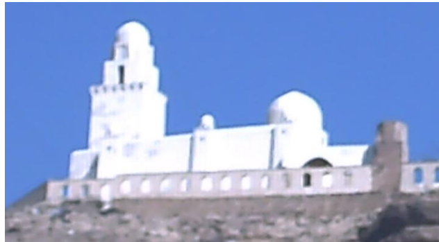
Fig. (116): Shows the defacement of the World Heritage property after renovating it by unprofessional people.
