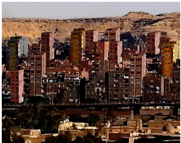
Fig. ( 207): Presents the researcher's vision for Manshiet Nasser after upgrading the buildings vertically using photoshop.
