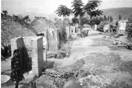
Figure 70: Basic latrine in each plot – incremental project, Visakhapatnum, India , 1988
