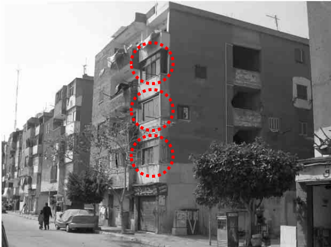
Figure 19: Closing the balcony is commonplace in governmental housing A photo from El-Zawia Elhamra- Cairo - Egypt
