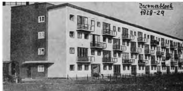
Figure 60: Housing complex, Frankfurt by A. Brenner, 1928–1929 Ref: Karel Teige. The minimum dwelling.
