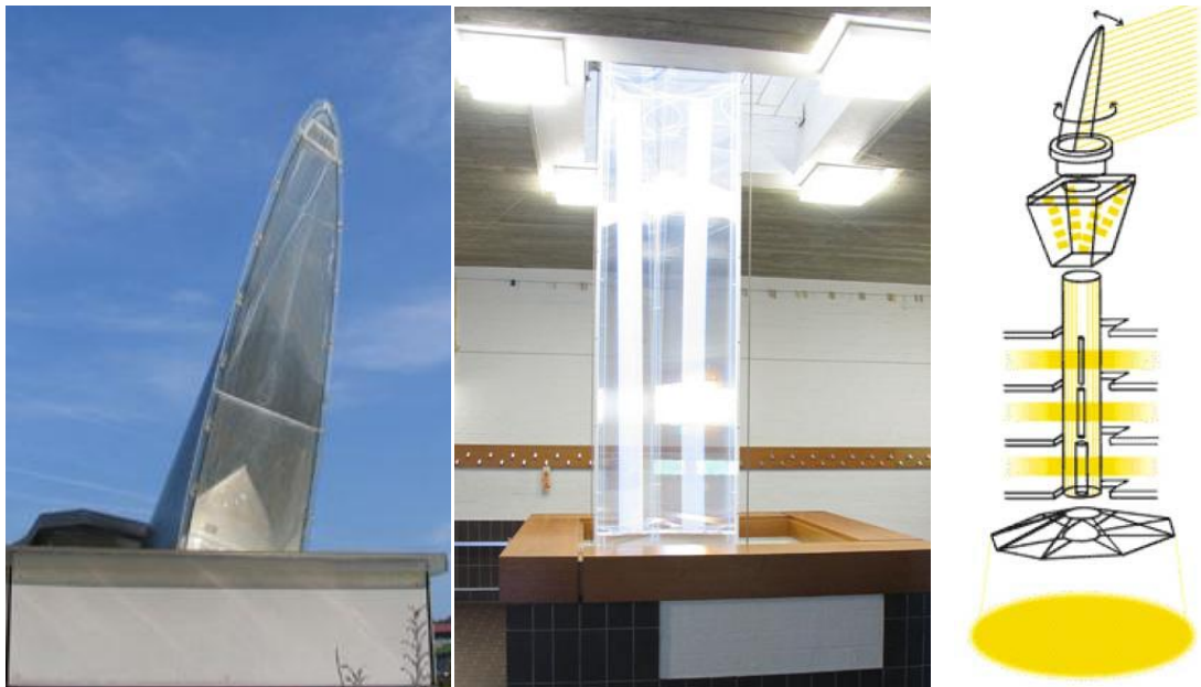
Figure 3.8: Heliobus collector (left); Heliobus light guide (middle); A schematic shows the heliostat, light guide including reflective diffusing extractors and an end diffuser (right).
