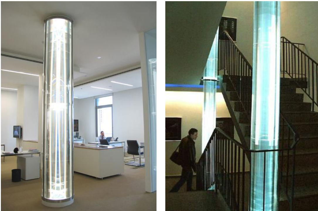
Figure 4.6: Vertical luminaires influence on working space (left) is more critical than its influence on public space such as stair cases (right)
