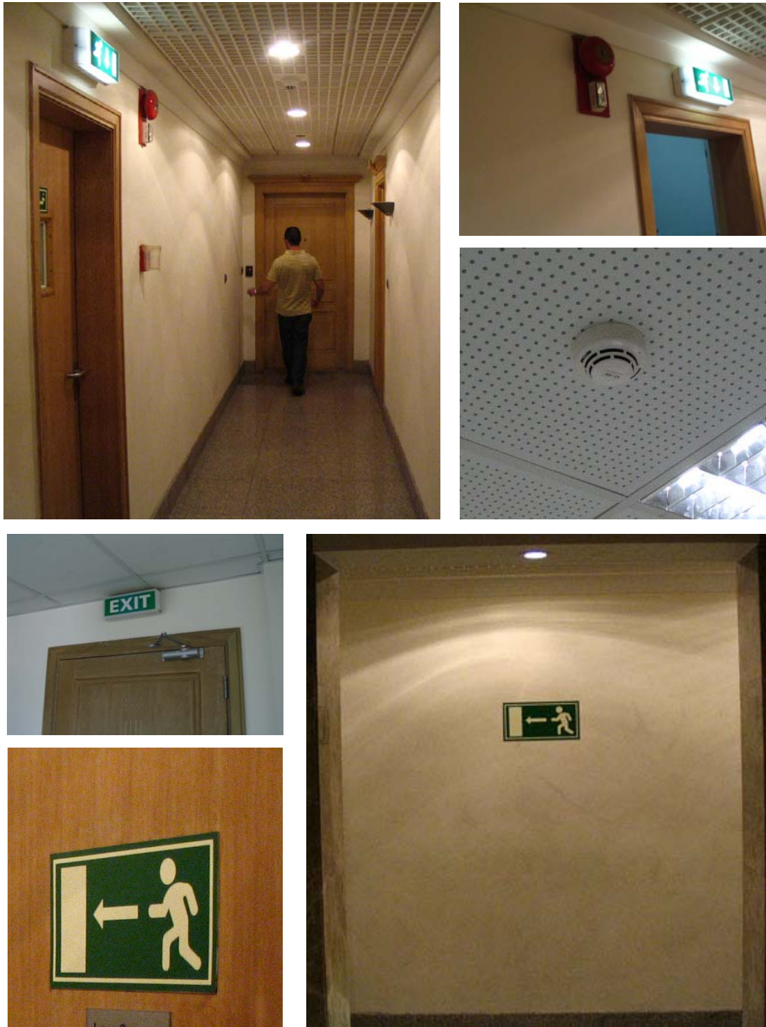
Fig. 7-8: Only a few signs for emergency exits could be found outside the office
