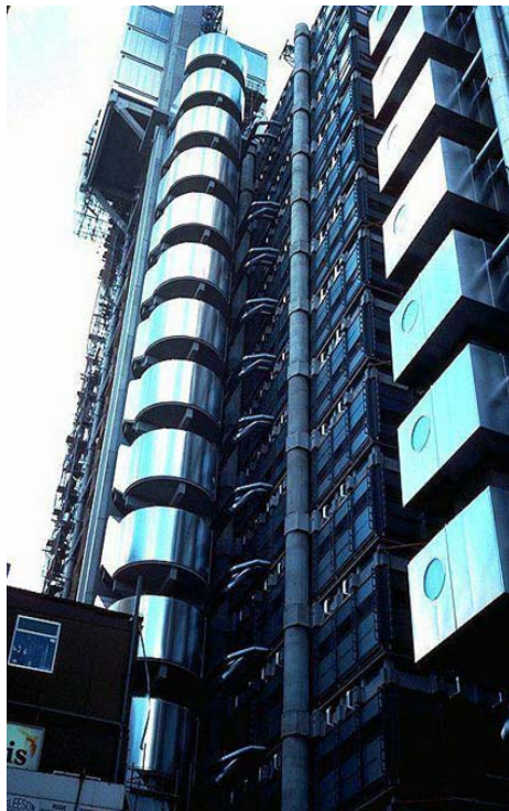
Fig. 1-6: Lloyds building, by Richard Rogers, London, UK. 1984
