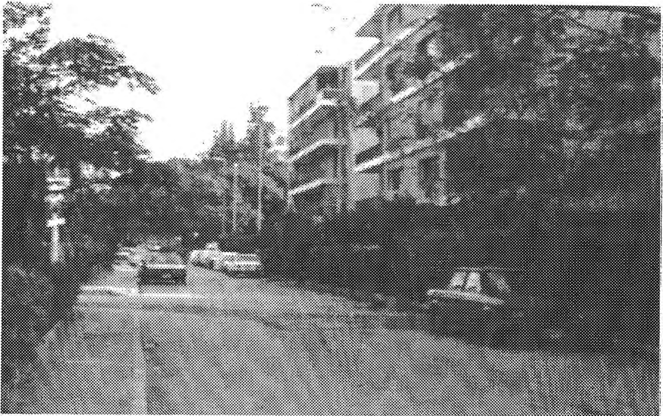
(Figure 4.29) Privatized Side Walks Used for Beautification in The Street Space B
