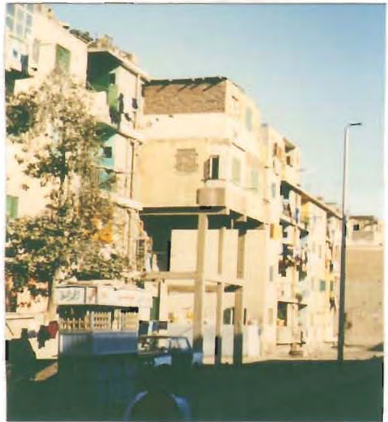
(Figure 3.3) Extensions of buildings taking place on marginal immediate spaces
