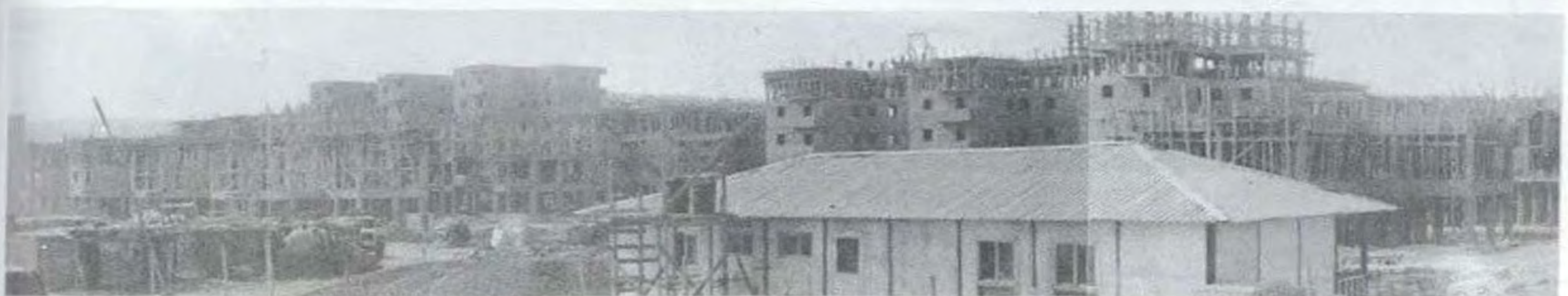
Fig.(37):The Mokattam Project; construction methods & stages (1)
