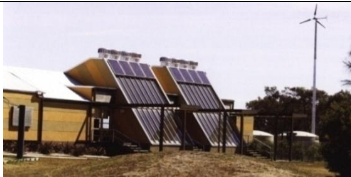
Figure 2. 43 Front façade at St Leonard's school, Sustainability centre. Solar chimneys provide heated air in winter and induce cross ventilation in summer. "Sustainable school book". 1
