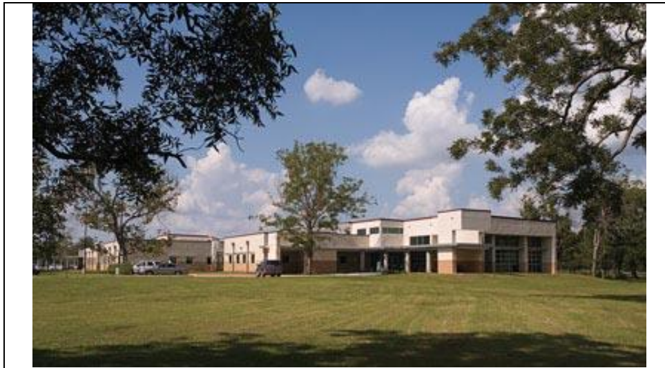
Figure 3. 51 The school building's dominant material is concrete masonry, which was chosen for its natural, durable quality. " Available:www.schooldesigns.com (Accessed 2009)".
