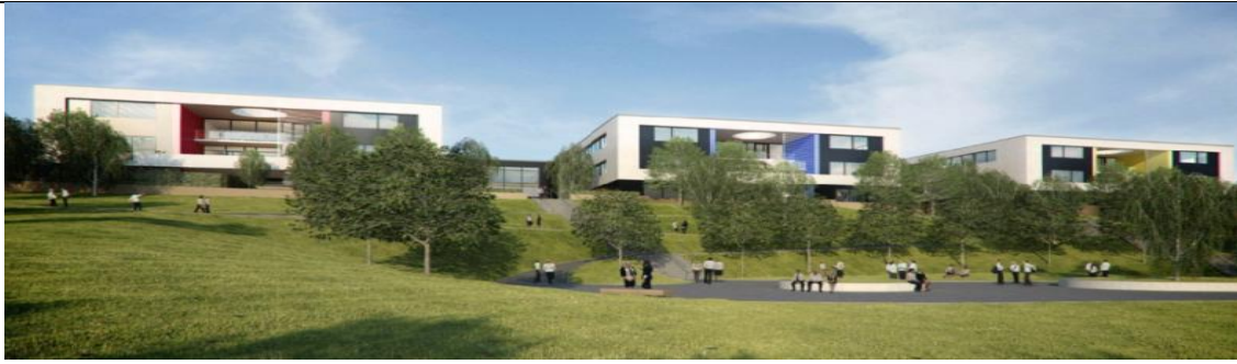
Figure 3. 41 Perspective from grounds- The scheme makes good use of its position giving views out across the landscape from the learning spaces (appropriateness).The three schools which make up the brief are carefully integrated yet retain their identities. “ http://www.cabe.org.uk/design-review/schools/successful-whole (Accessed2008)”.
