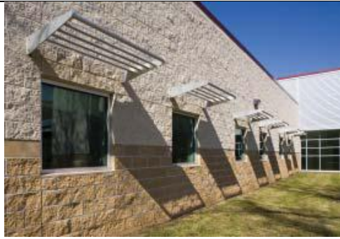
Figure 3.47-Aluminum shading outside the building reduces heat load on the windows, minimizing cooling needs inside, and the shades were “low-cost items that get big gains” financially, according to Henry. Available:www.greenrightnow.com (Accessed 2009)”.
