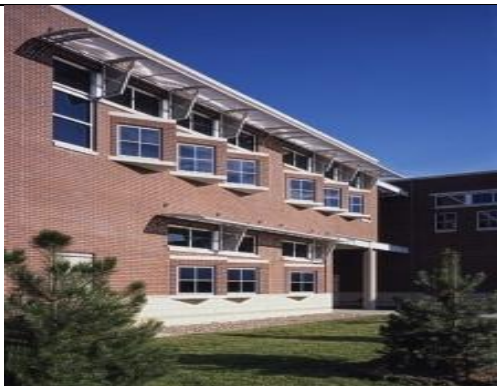
Figure 4.55 These articulated windows and exterior window coverings allow maximum daylight into the building while minimizing the amount of direct sunlight. ."Sustainable School Book". 5
