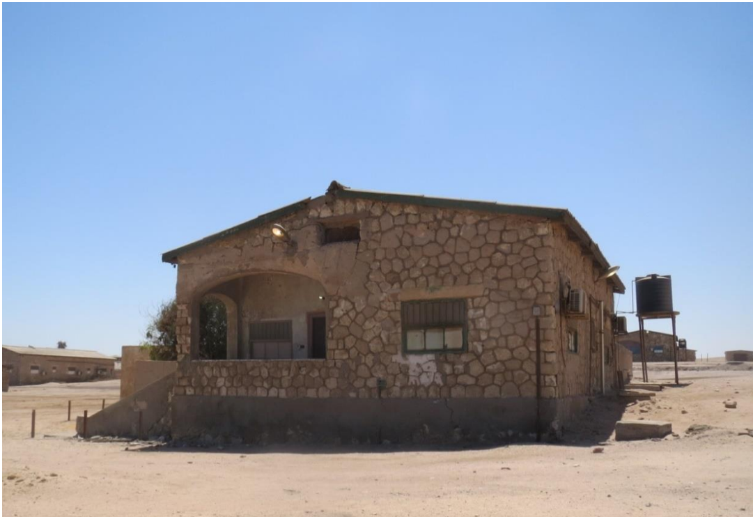
Figure 16 Ras Gharib Southern Area Housing (Source: Kosta Mathey)
