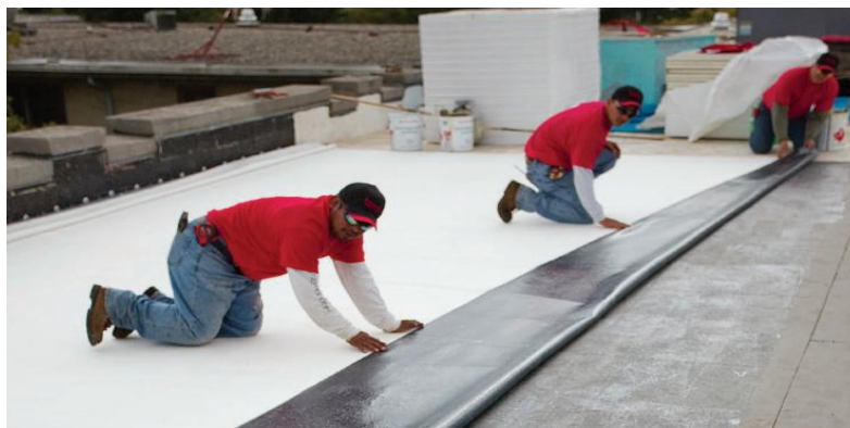
Figure 4.28 Installation of EPDM membrane on the roof
