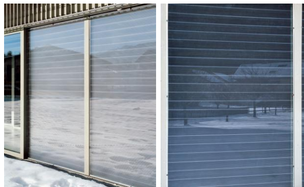
Figure 4.9 outside detail of latent heat-storing facade, uncharged state (opaque). Detail of latent heat-storing facade, charged state (translucent).
