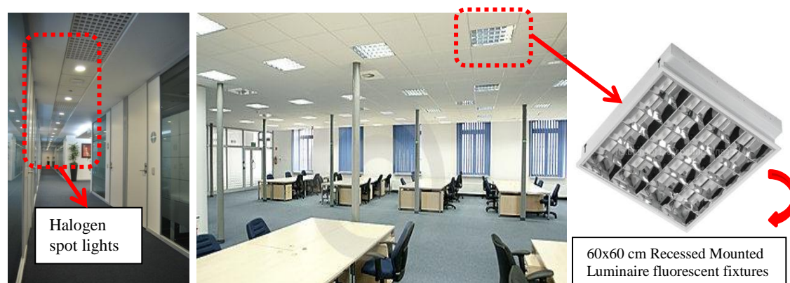
Figure 5.22 Light fixtures used in the office space and corridors. Source: URL: http://www.smart-villages.com/en/brochure/page/179/type/2 , accessed June 22, 2013.
