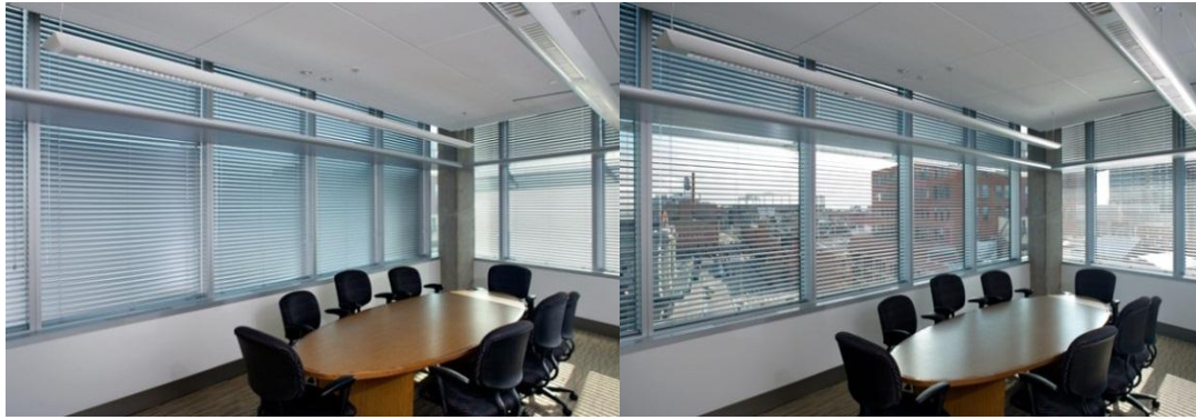
Figure 4.15 Horizontal window blinds in a meeting room.
