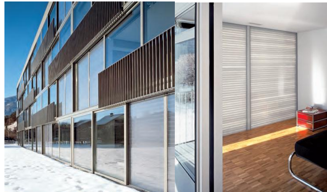
Figure 4.8 Senior citizens' apartments: view of south facade. Side view of south facade. Inside view of latent heat-storing facade.
