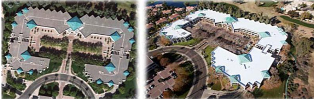
Figure 4.27 Scottsdale Insurance Company before and after cool roof installation
