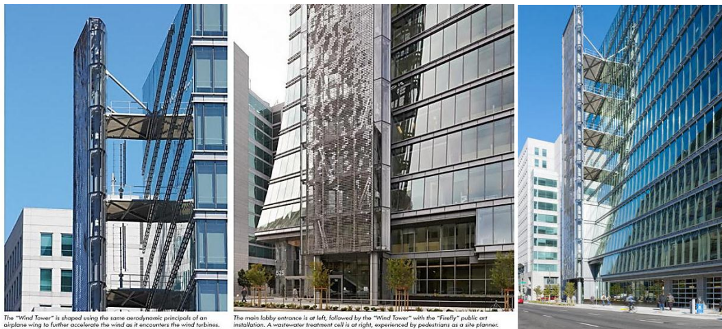
Figure 4.42 View of the Wind Tower form the side and Wind Tower with the Firefly installation
