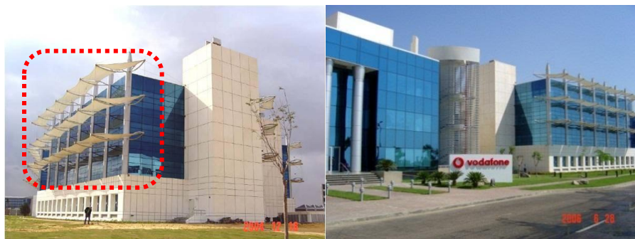
Figure 5.19 Three row of horizontal membranes stretched between steel posts stabilized by a net of vertical, horizontal and bracing cables.
