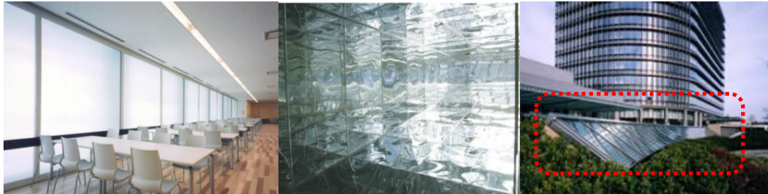
Figure 4.37 Left : Photo of cafeteria brightly lit by mirror duct. Middle : Interior photo of mirror duct. Right : Light collection part of mirror duct.
