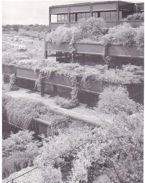
Fig.4-13: The gateway house at Basingstoke built in 1977, picture taken in 1986
