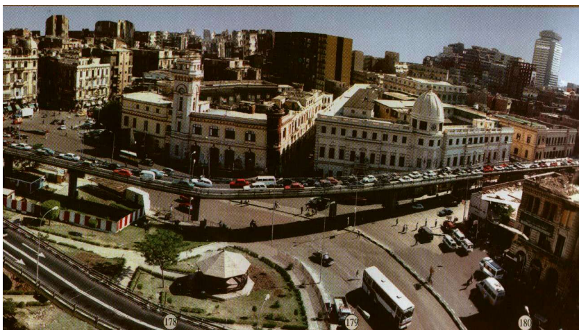
Figure 4.94. Al-Azhar bridge (source: www.urbanharmony.org ).
