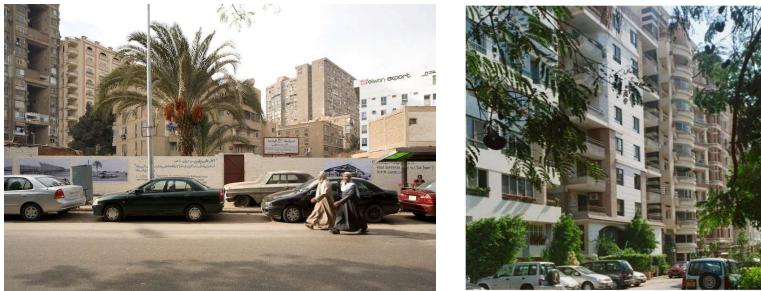
Figure 4.47. Skyscrapers located in Maadi Corniche (source: http://www.panoramio.com ).
