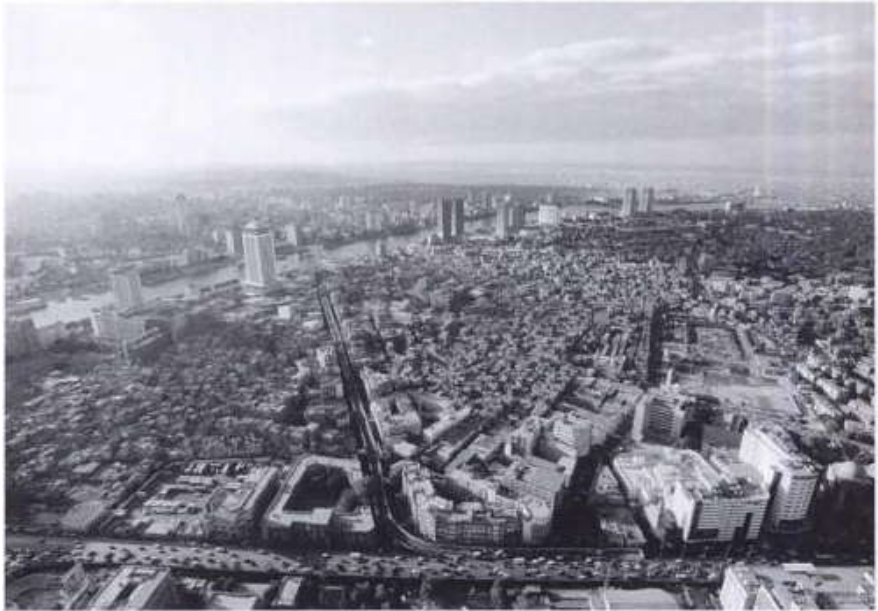
Figure 4.93. 6 October bridge ( source: Golia, 2004).
