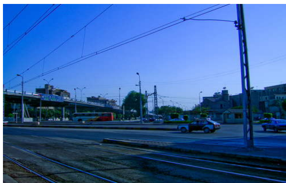
Figure 4.21. El-Galaa bridge as an overhead edge (source: http://www.panoramio.com ).
