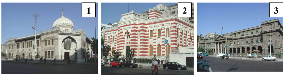
Figure 4.106. Remarkable buildings of Ramsis street, Cairo CBD (source: www.cultnat.org ).
