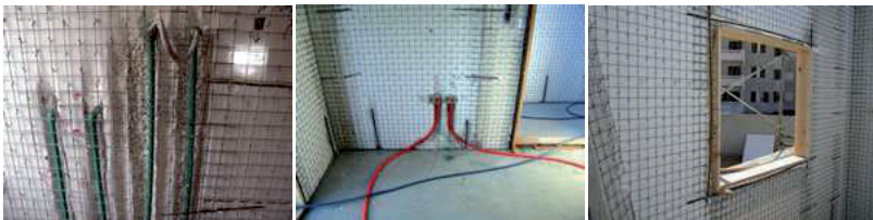
Figure (5.31) Reinforced foam panels “Thermal Insulation” with piping & wooden works (Tridipanel, 2010)
