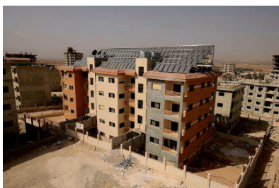
Figure (3.4) Photovoltaic Panels, Syria (Med-Eneec, 2010)
