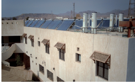
Figure (4.22) Sharm el Sheikh, students residential building (Med-Eneec, 2010)
