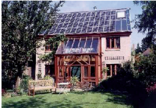
Figure (4.1) Oxford eco-house, UK (Roaf, 2001)
