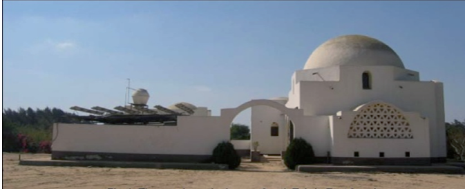
Figure (4.20) The passive solar house, South Tahrir, East facade and photovoltaic panels. (DDC, 2006)
