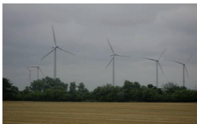
Figure (5.3) Wind energy, Red Sea, Egypt
