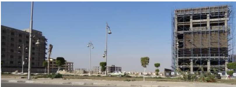
Fig. 20: Picture of the project location
